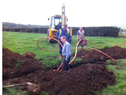
Multicore ducts being moleploughed under a road by Tom, and Robert Brian and Phil helping John get it through.
