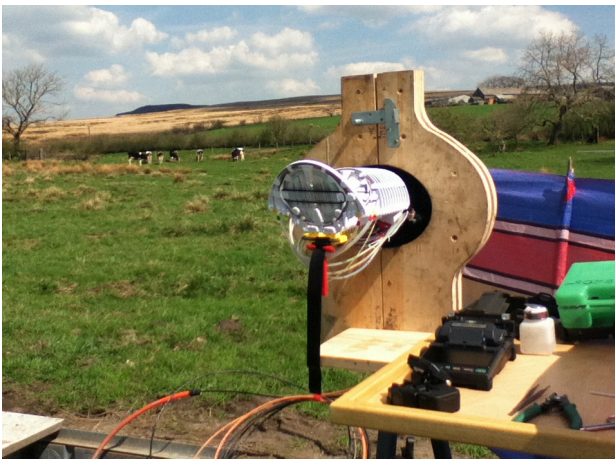
A sunny fusing day fusing the fibre where the Quernmore and Abbeystead routes join below Jubilee Tower.
