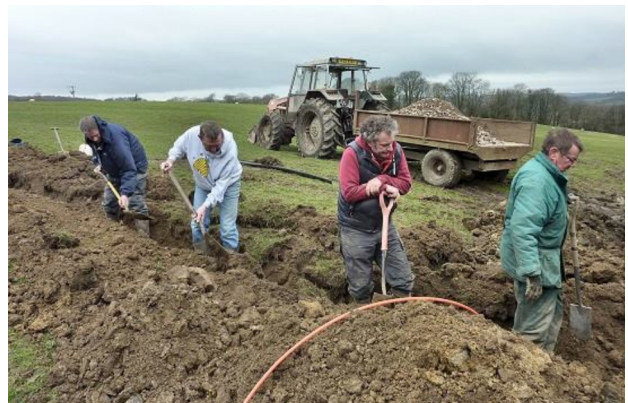
Bobbiners levelling the trench.
