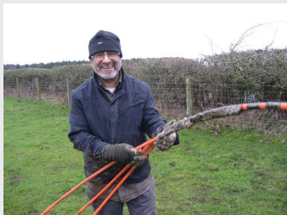
Sam putting the ducts in the trenches.
