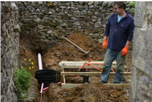
Phil Stone setting the ducts into the chamber next to the plinth.
