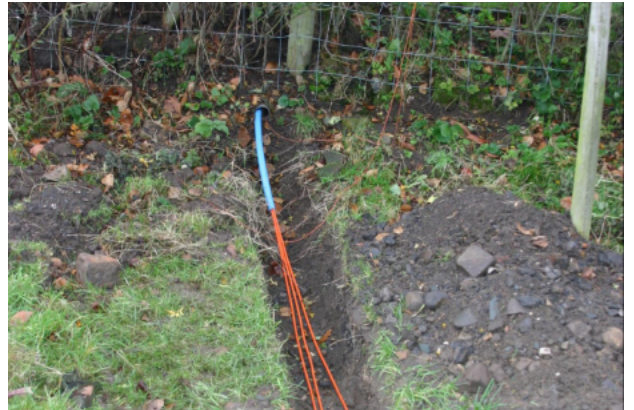
Sub-ducted ducts under walls and fences.
