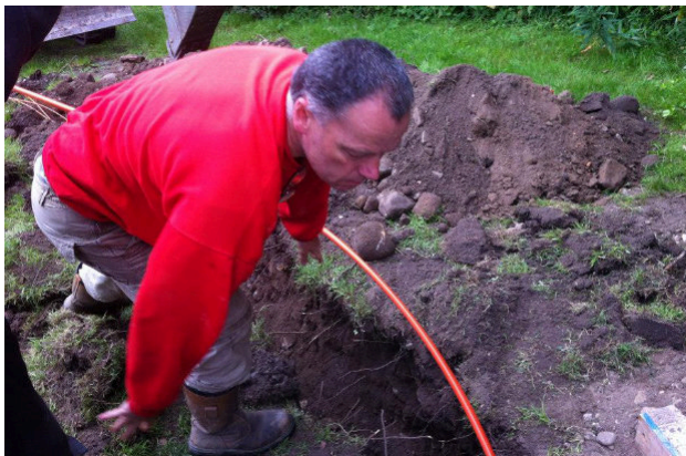
Carl Hunter in the trenches laying duct.
