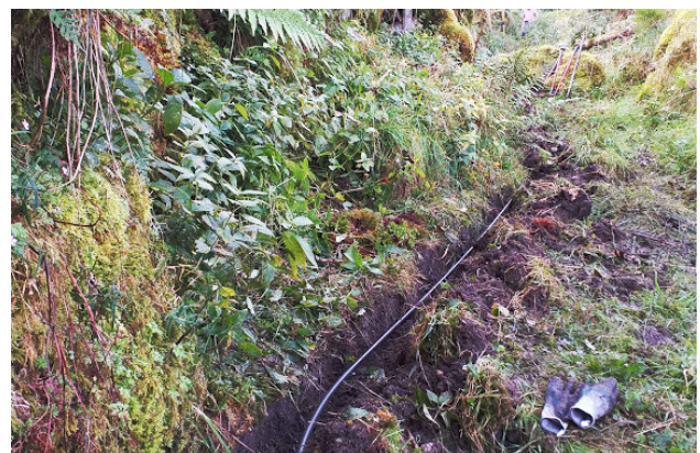
Black 18mm duct used for extra protection through limestone.
