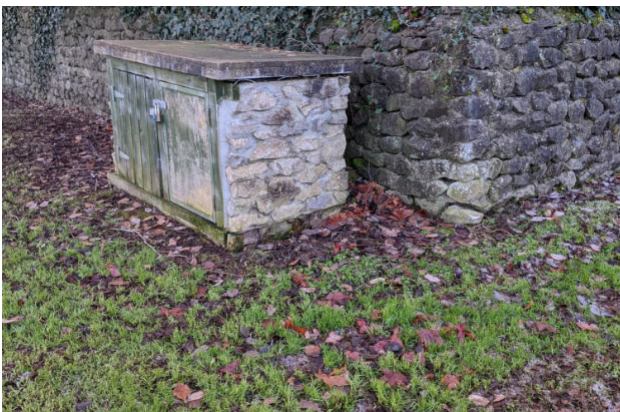
Carl builds our own electric cabinet to match the stone wall.
