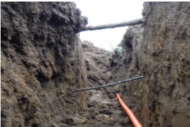
Digging under utility cables.
