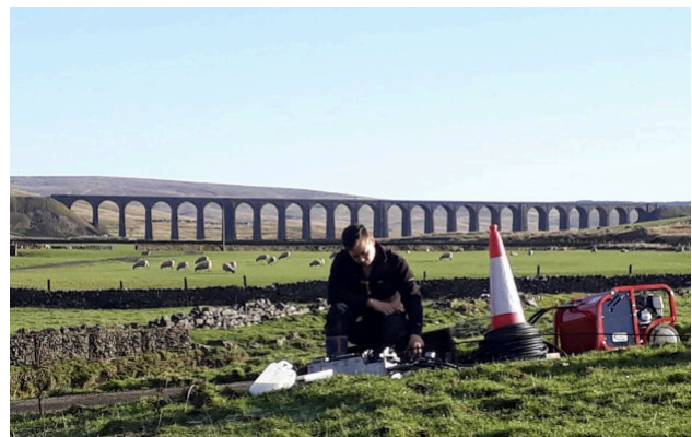
Sam Robson from B4RN civils, blowing the Ribbleshead fibre.
