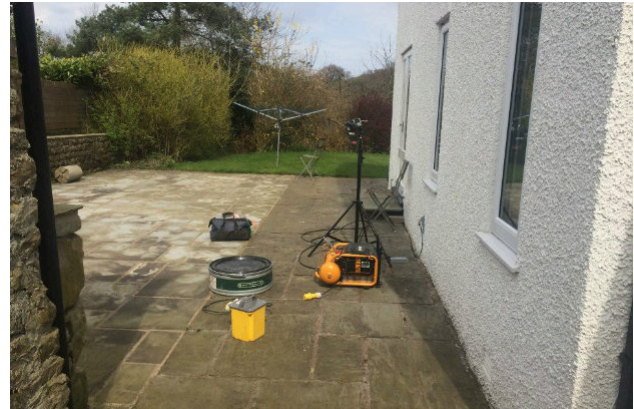
Blowing the house fibres.
