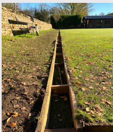
Replacement of the guttering around the village bowling green.
