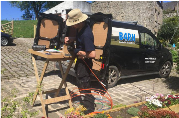
Paul fusing a small bullet join.
