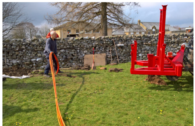
Ray Newport from Dent comes to lend a hand with the mole plough.
