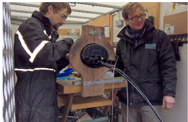
Joe Brown and Simon Done fusing the main core.
