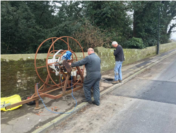
Tommy and Dave Connor winching the duct over the bridge.
