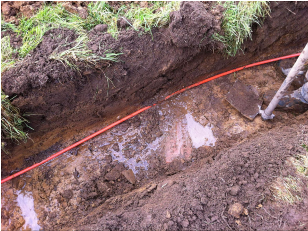
Mains electric found and carefully excavated around it.
