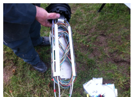
The tubes not split are coiled below.
