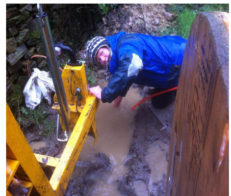
Nicky Abraham pulling the duct through a chamber.
