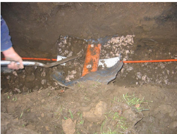
Duct going under a drain.
