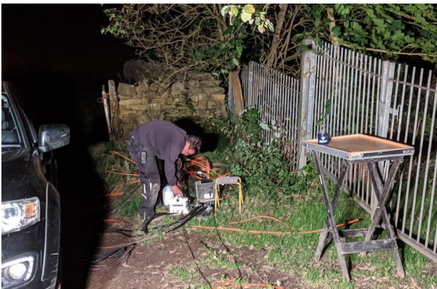
James re-blowing new fibre.
