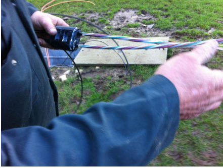
Outer sheath of the fibre removed.
