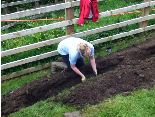
Putting soft fill on the duct.
