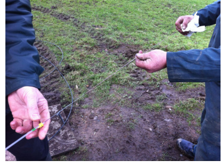
Tube sheath of the fibre removed.
