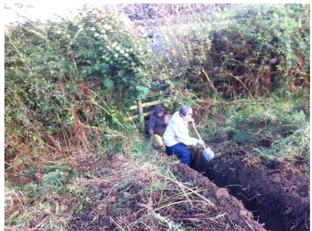
Harry and Sue Ball levelling out the bottom of the trench under the hedge
