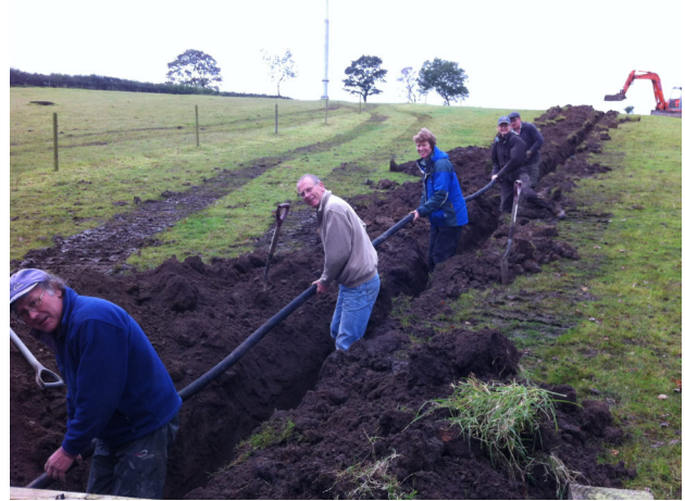
Volunteers laying drains, utility ducts and B4RN duct in the trench.
