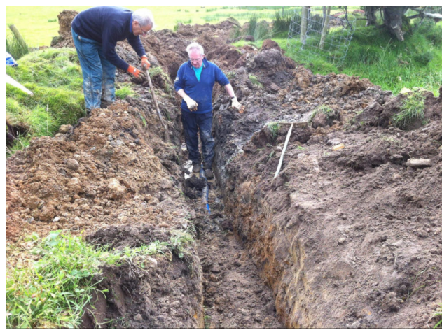
Iain helping in a tricky area, using alkathene pipe for extra protection.
