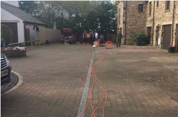
Laying out the new ducts.
