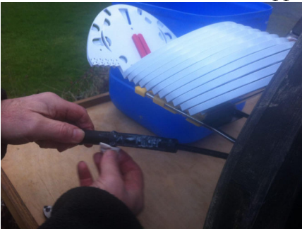
Lubricating the grommet that holds the fibres/duct.
