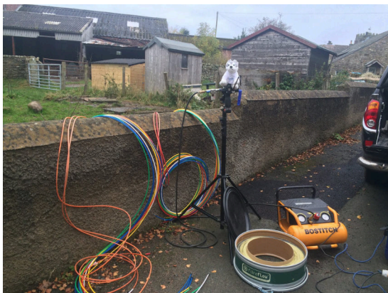
The customer tubes getting their fibre blown.
