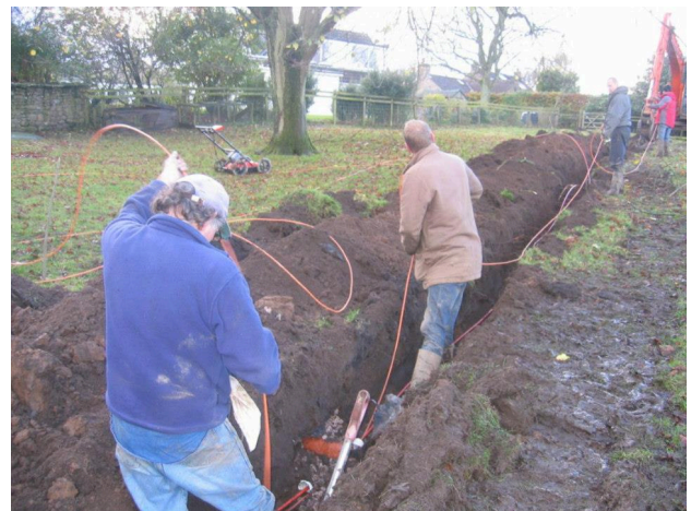
Chris Hall and Eric Lange going under drains following the digger.
