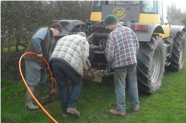
Feeding the duct into the mole plough.
