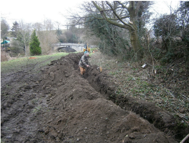
Backfilling the trench with soft fill.
