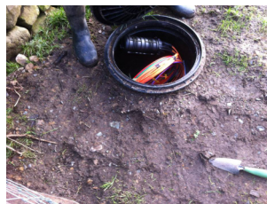
Round chamber with bullet, oblong chamber with 20 metres of fibre in it.
