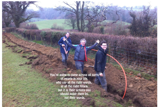
Bobbiners laying duct in the trench.
