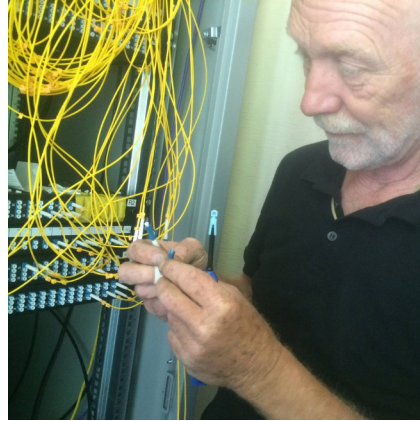
Bruce cleaning the patch leads to connect new customers in the cabinet.
