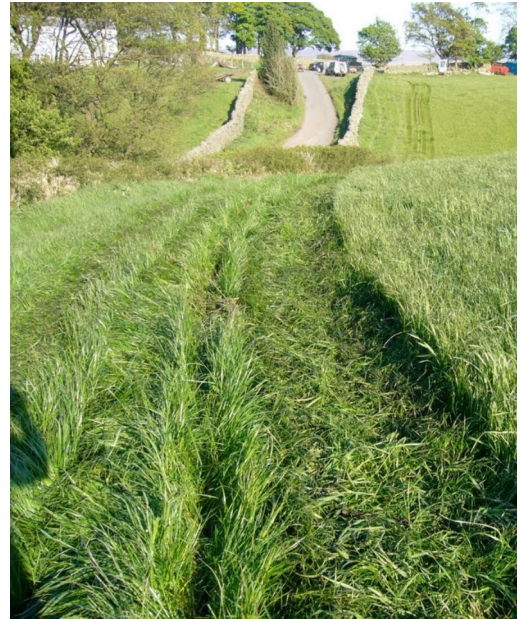
The 800 metre mole plough, the first done by a rural altnet.
