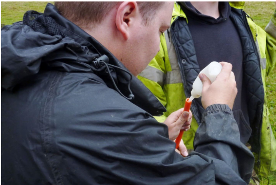
Alistair, putting the lubricant into the duct.
