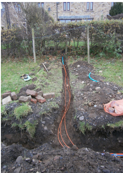
Splitting ducts off from the multicore into houses.
