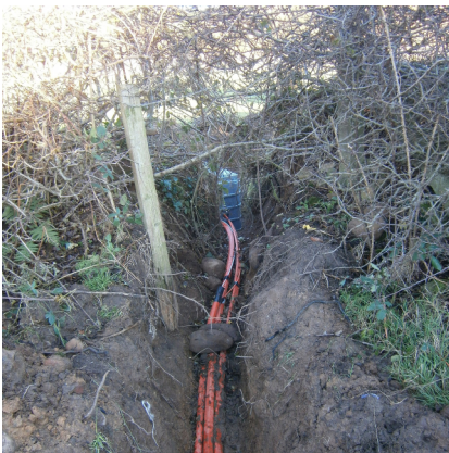
Several multicore ducts going under a fence.
