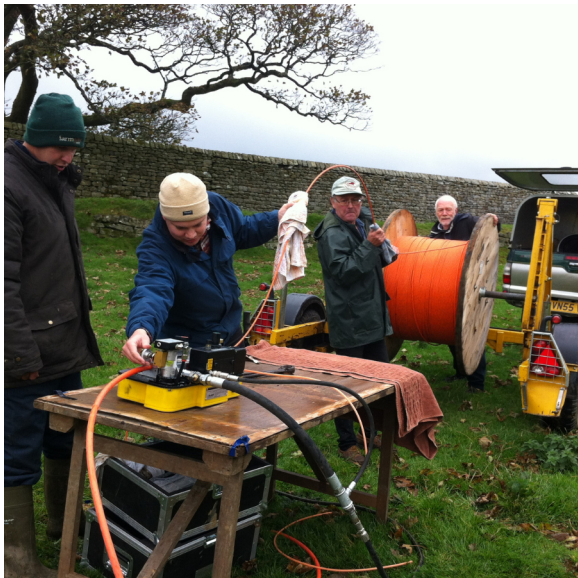
Alistair blowing the fibre over Littledale.
