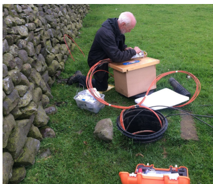
Bruce fusing customer fibres into a bullet.
