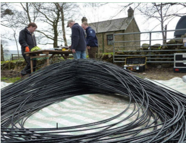
Alistair and Bruce blowing core fibre at Eileen's farm in Abbeystead, 17th May 2013.
