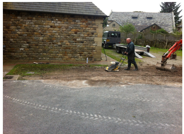
Trench filled in, and Tom whacking it down level.
