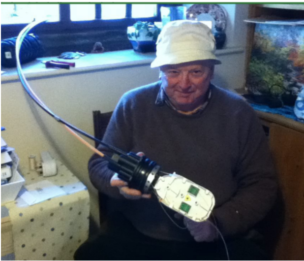
Walter holding a small bullet (an FST) which was fused in the house due to the high winds and dust outside.
