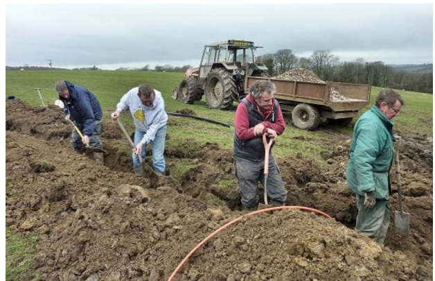
Bobbiners levelling the trench.
