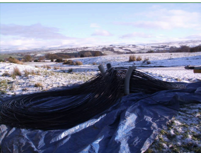
Fleeting fibre on the way from Wray to Thrushgill and Lowgill.
