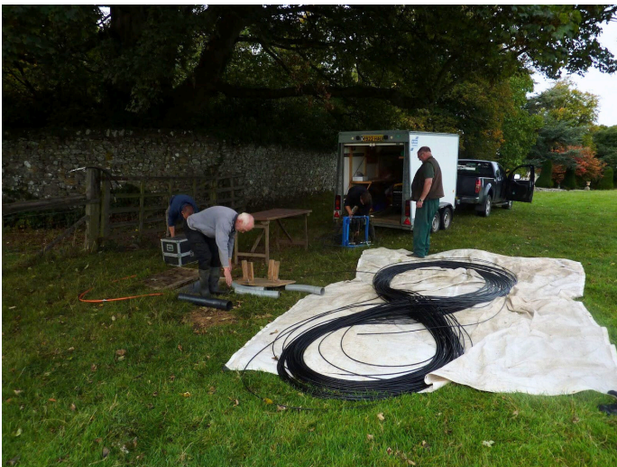
Fibre fleeted onto a tarpaulin to keep it clean.
