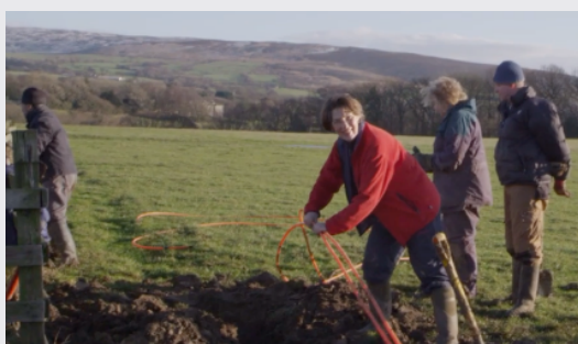
AnnaGerd putting the ducts in the trenches.
