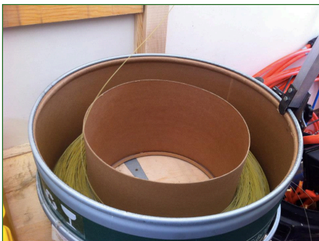
House fibre being blown from the pan.
