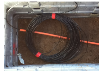
Round chamber with bullet, oblong chamber with 20 metres of fibre in it.
