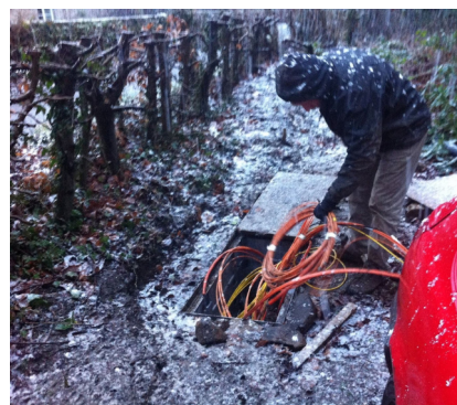
All weathers: Bruce getting customer ducts out of the chamber ready to blow fibre in.
