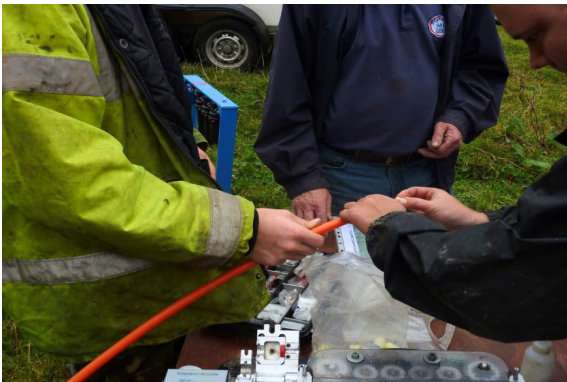
Putting the sponge into the duct.
