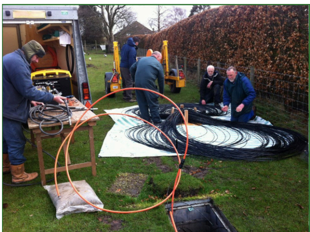
Frank Balassa and Chas Lee join Bruce and Tom blowing fibre from Quernmore to Abbeystead.
