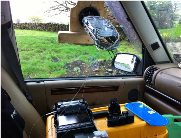
Fusing Eileen's bullet with the FRBU holder jammed in the car window to keep dry.
