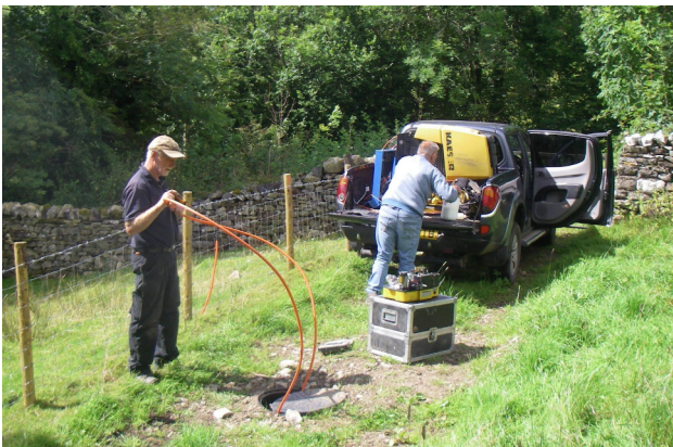
Bruce Alexander and Frank Brown blowing core fibre.
