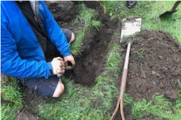
Tony Middleton digging for a duct dent.
