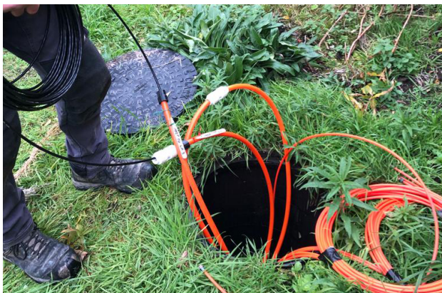
Bruce blowing core fibre.
