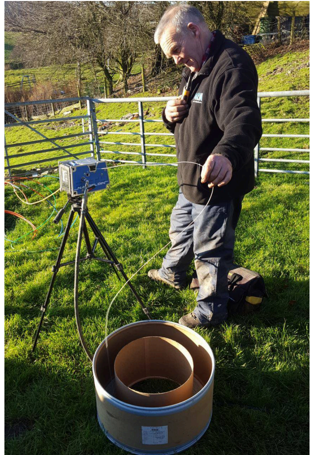
Frank feeding house fibre into the blower.
