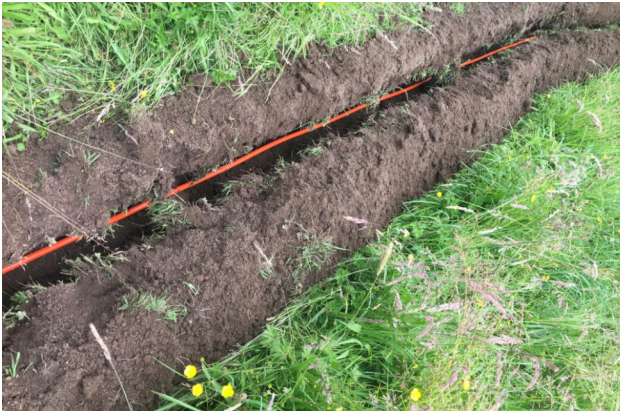
Laying the duct in the trench.
