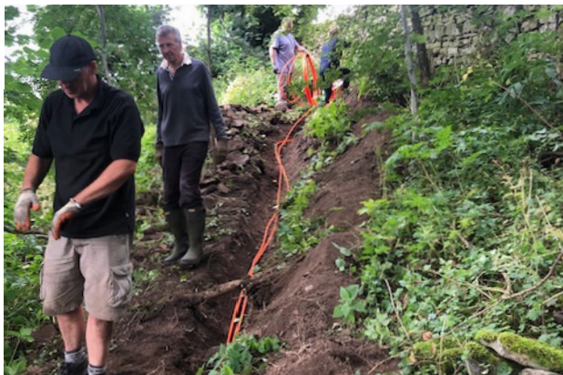
Laying the ducts in the trench.
