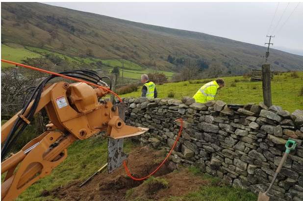
The mole with the duct ready to thread under the wall.
