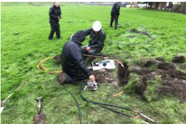
Fleeting out the fibre from the blockage.
