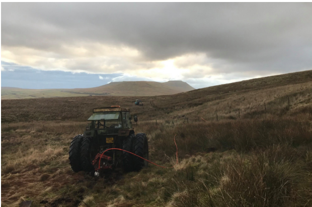
Moleing the duct over the tough fell.
