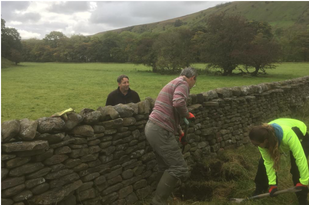
John Colton digging under a wall for the duct to go through.
