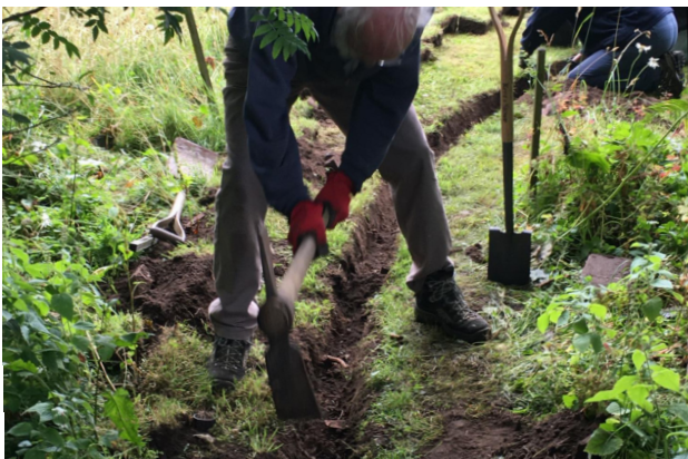
Pick axes and mattocks to get the trenches dug.
