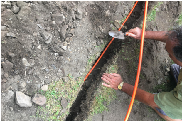
Soft backfill on the duct.
