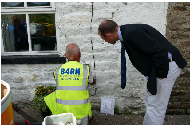
Matt watches Barry blowing a house fibre.
