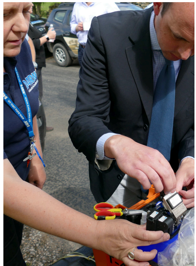
Jorj Haston showing Matt how to fuse the house fibre.
