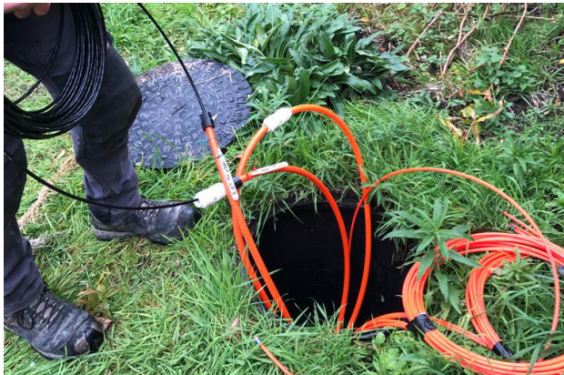
Bruce blowing core fibre.
