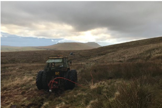
Moleing the duct over the tough fell.
