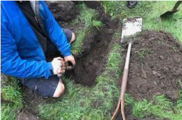
Tony Middleton digging for a duct dent.
