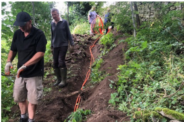
Laying the ducts in the trench.
