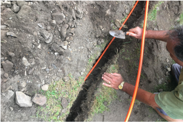
Soft backfill on the duct.
