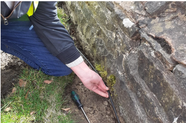
Fixing the external house duct to the wall.
