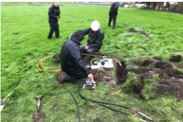
Fleeting out the fibre from the blockage.
