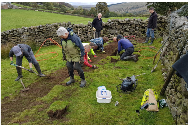
Volunteers backfilling the trench over the duct that has gone under wall.
