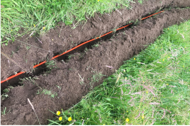
Laying the duct in the trench.
