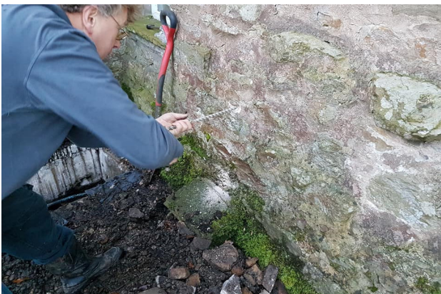
Philip drilling the wall for the outside box.
