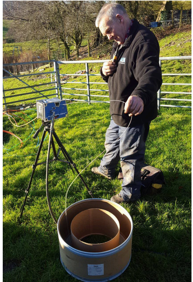
Frank feeding house fibre into the blower.
