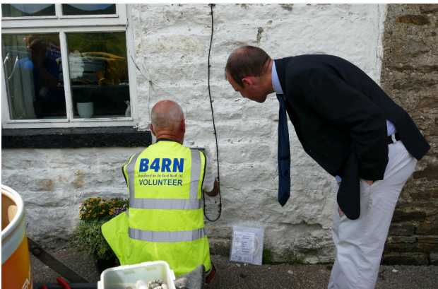
Matt watches Barry blowing a house fibre.
