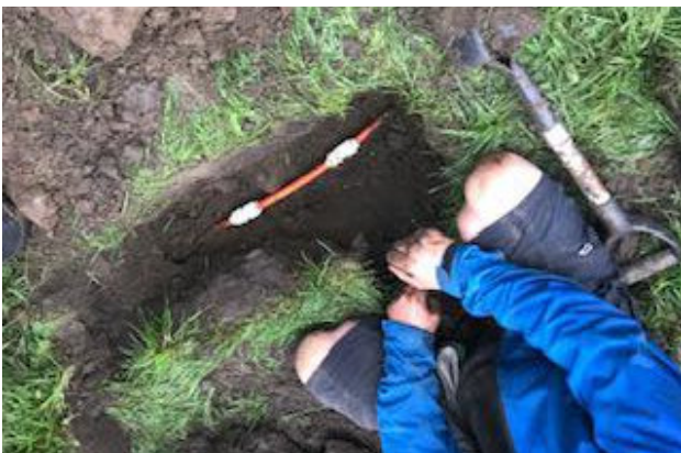
Finished job with a little patch jointed on.
