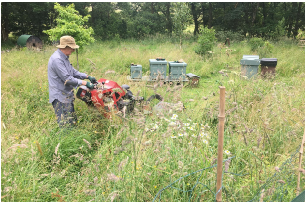
Trenching through a long rough stretch, lots of bees, so no diggers.
