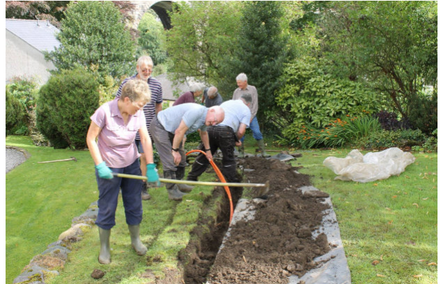
Laying the duct in a trench and backfilling.
