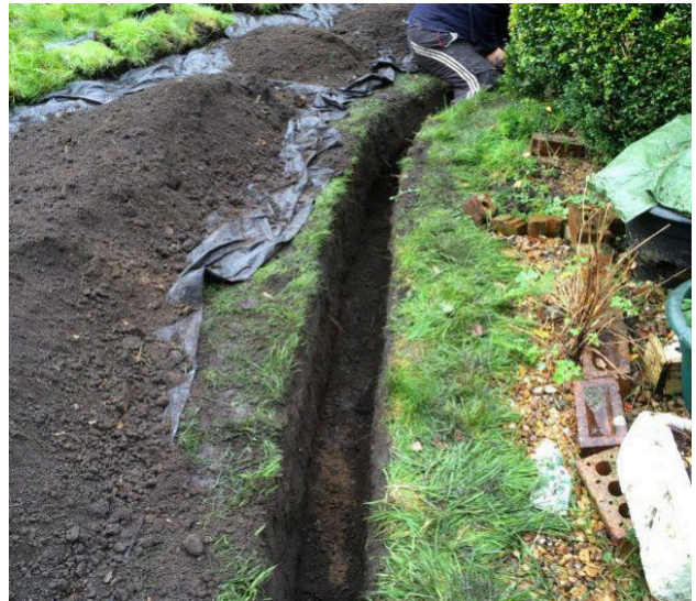
Digging the garden trench with soil put onto a sheet.
