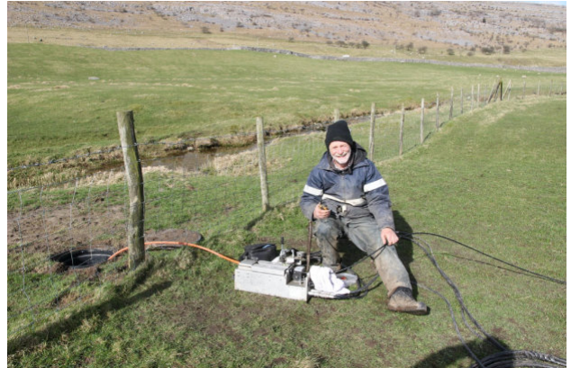
Bruce blowing core fibre.
