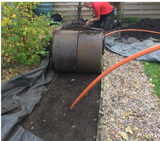
Rolling the trench level.
