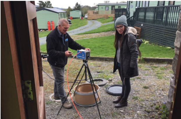
Frank blowing fibre to the caravans, and talking to Kira Allmann.
