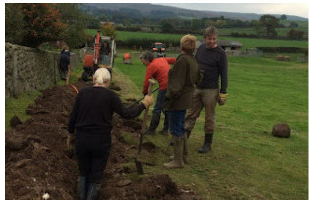
Frank digging, and the volunteers lay the duct and soft fill.
