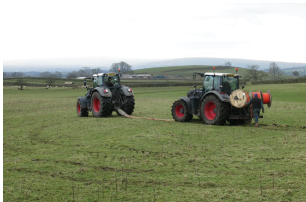
Sometimes they used two tractors to pull the mole plough.
