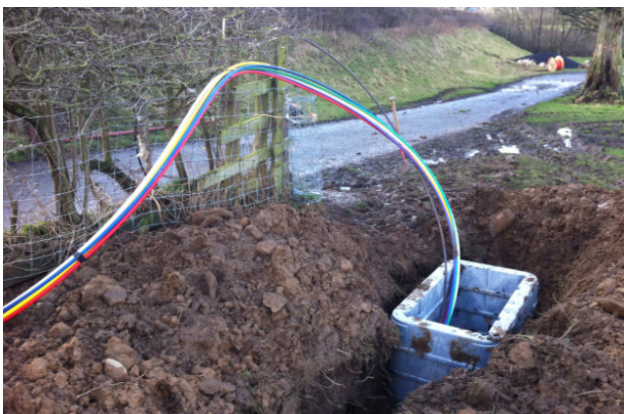
Multicore duct and the last chamber in Wray before the railway line.
