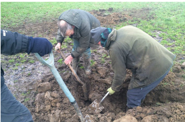
Frank was handy with a spade where two stones had crushed the duct.
