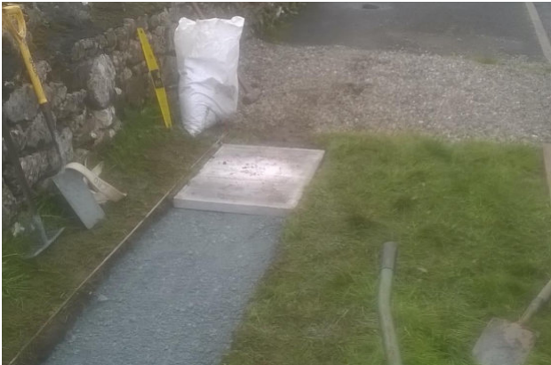
Duct laid in the verge and covered in gravel.
