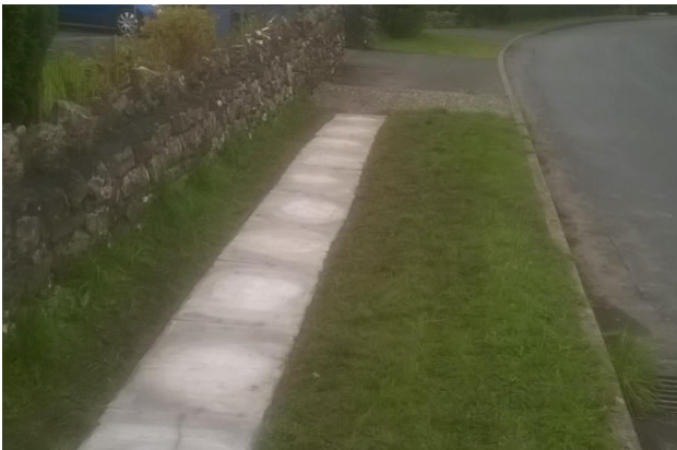
Paving stones on the gravel over the duct.
