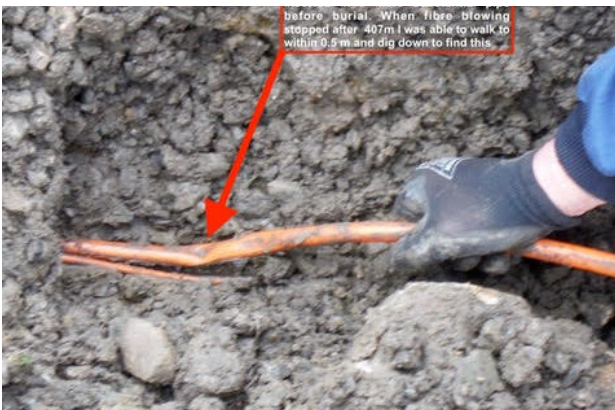
Duct crushed by two big stones.
