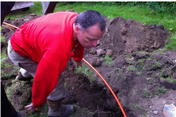
Carl Hunter in the trenches laying duct.
