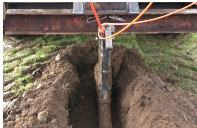
Starting the mole plough from a trench.
