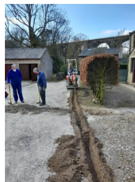
Trenching with a mini digger and sub-ducting with alkathene pipe.
