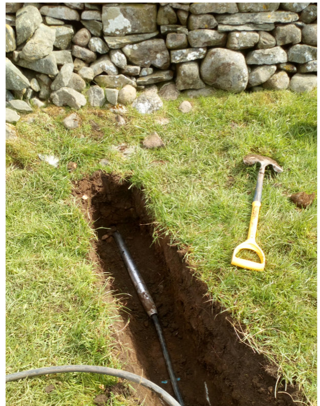
The mole ready to go under the wall.
