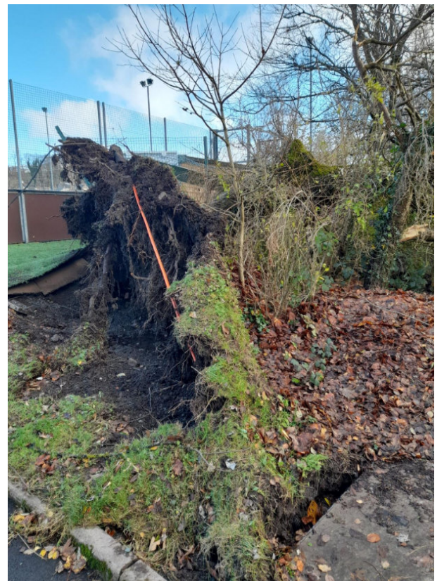
The duct pulled up in tree roots.
