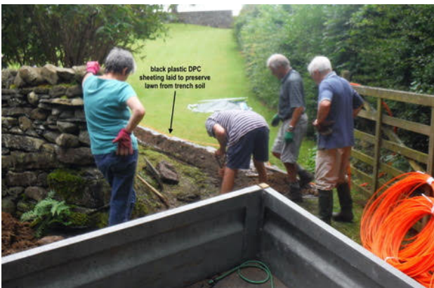
Black sheet laid to protect lawn from trench soil.
