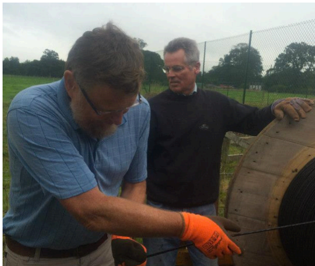
Feeding the fibre off the reel into the blowing machine.
