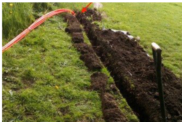
Multiple ducts being buried, each one of them a separate branch.
