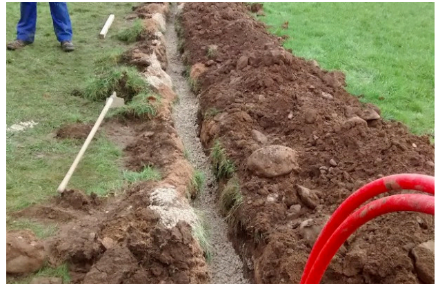
The electricity trench.
