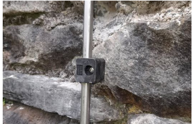
Stainless steel pipe, firmly secured with fibre duct inside.
