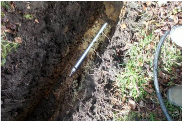
The mole comes out at the other side of the wall.
