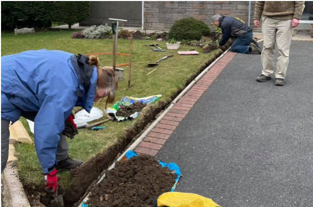
The house digs in progress, from the toby box to the property.
