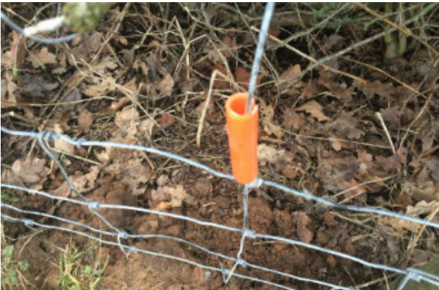
A small piece of split gash duct on the fence so the farmer knows where not to knock a post in.
