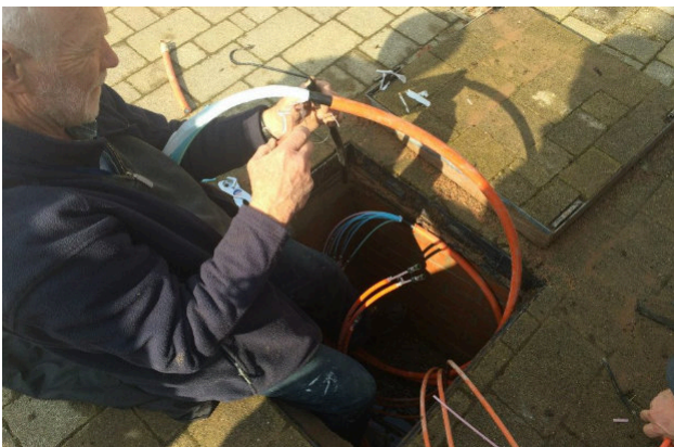
Bruce coupling up the spaghetti to blow fibre to the customers.
