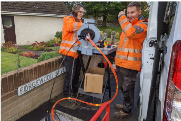
Alex Colton and Kit Mackereth fusing at a pavement chamber.
