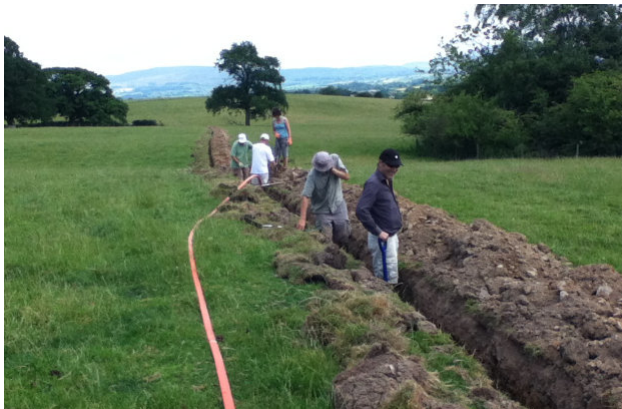
Volunteers laying the duct and backfilling with soft fill.
