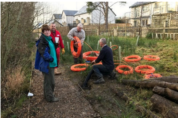
Duct measured out to reach each property from a chamber.
