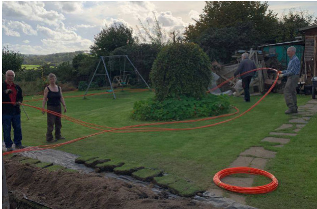
Laying out duct to properties.
