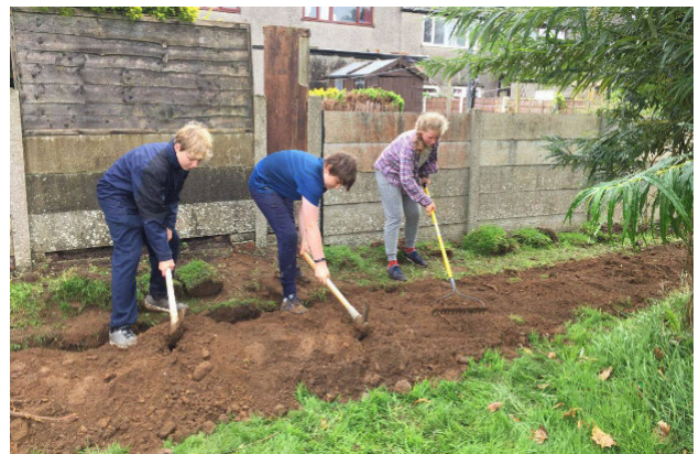
Backfilling the trench with soft fill.
