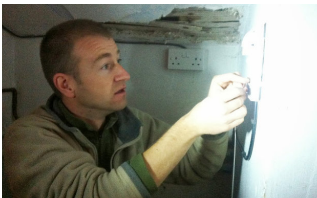
John Hamlett fusing customer connections.
