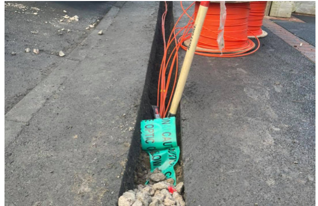
Multiple ducts in the trench, marker tape and clean fill.
