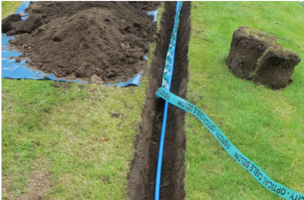
Garden sub-ducted in alkathene with metallic tracer tape.
