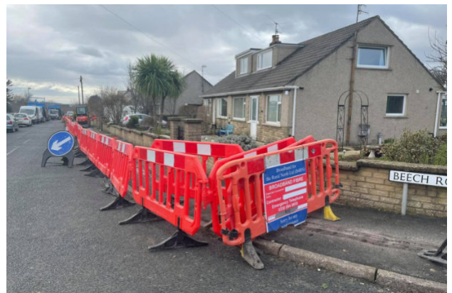
Small sections barricaded each day to minimise disruption.
