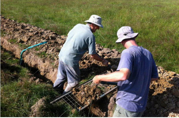
Peter Docton and John backfilling with sieved soil to get stones out.
