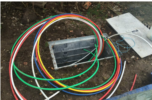
Lots of multicore duct was laid to enable Halton to join on.
