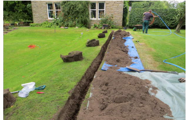
A long neat garden dig, with spoil kept off the lawn surface.
