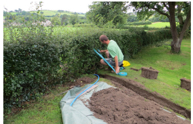
John digging under a hedge and threading duct through alkathene pipe.
