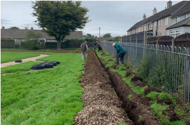
Soft fill going onto the duct in the trench.
