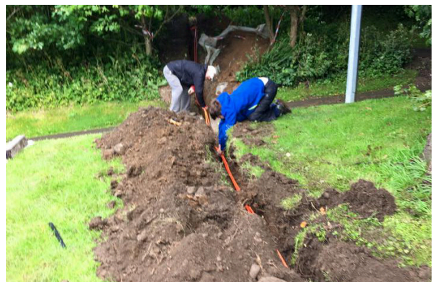
Laying duct in a trench prior to backfilling,
