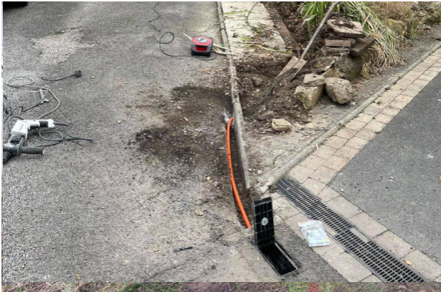
This is what the small toby box in the pavement looks like.
