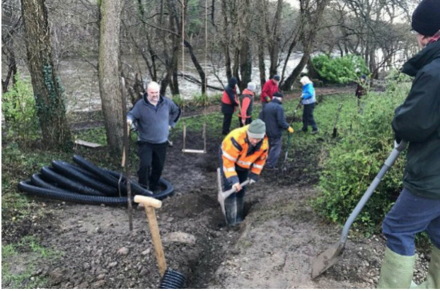
Volunteers laying sub-ducting through a rough area.
