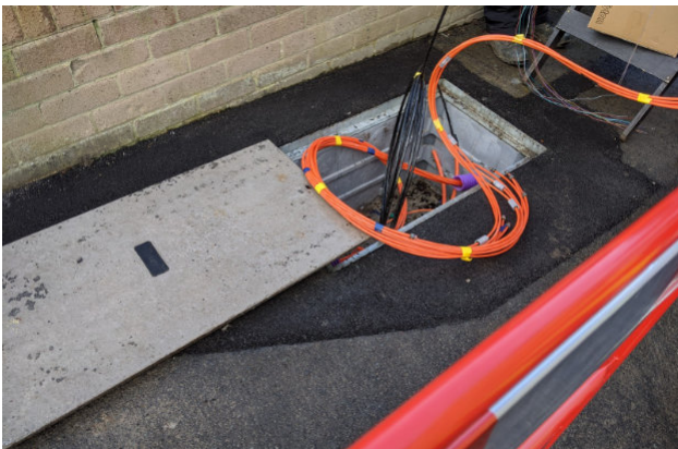
The B4RN chambers. Customer duct is orange, the fibre is black.
