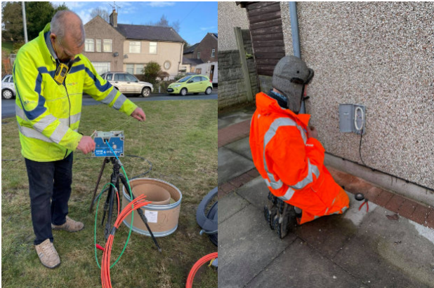
Frank and Barrie blowing the house fibres.
