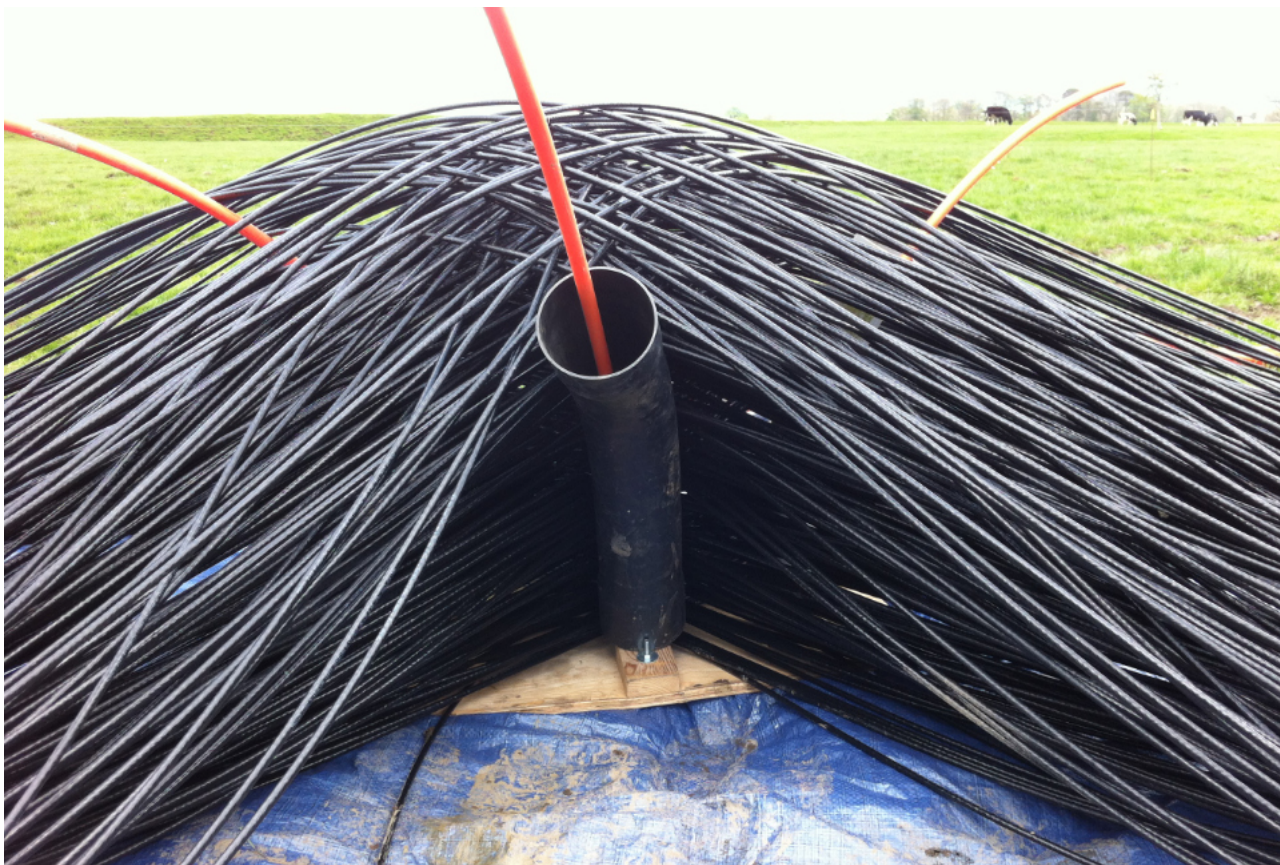
Using bits of duct to extend the drainpipe arms of the fleeting table.
