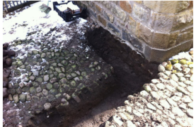
Cobble mining to get the connection to old estate houses.
