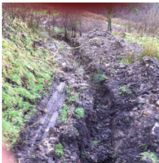
George did not backfill his trench totally until the blow was complete in case they had to dig down to a bend or a blockage.
