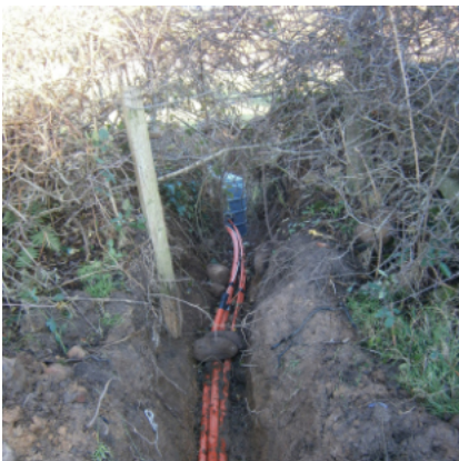
Several multicore ducts going under a fence.
