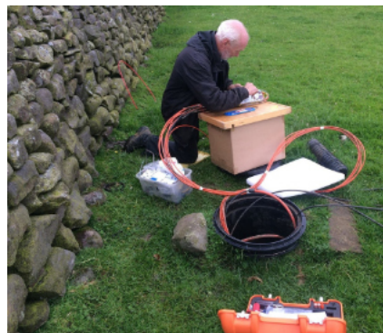
Bruce fusing customer fibres into a bullet.
