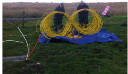
Final fleet, and turning the fleet before starting the blow again.
