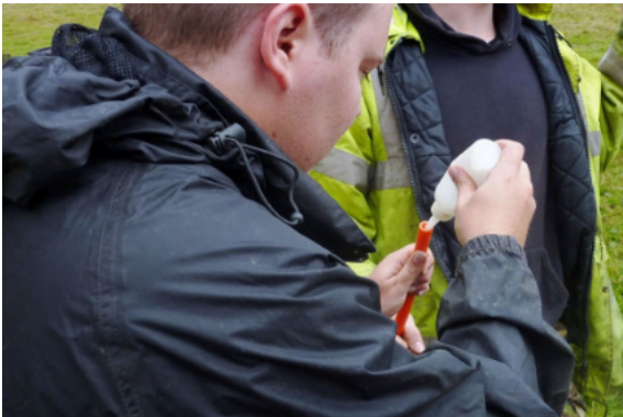
Alistair, putting the lubricant into the duct.
