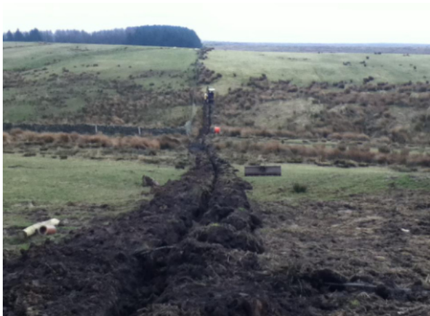
Joining the route from Quernmore to Abbeystead. Zoom in to see how shallow the BT phone lines are buried, we have to go under them.
