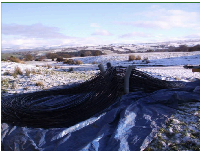
Fleeting fibre on the way from Wray to Thrushgill and Lowgill.
