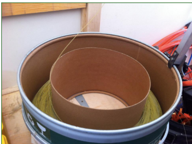
House fibre being blown from the pan.
