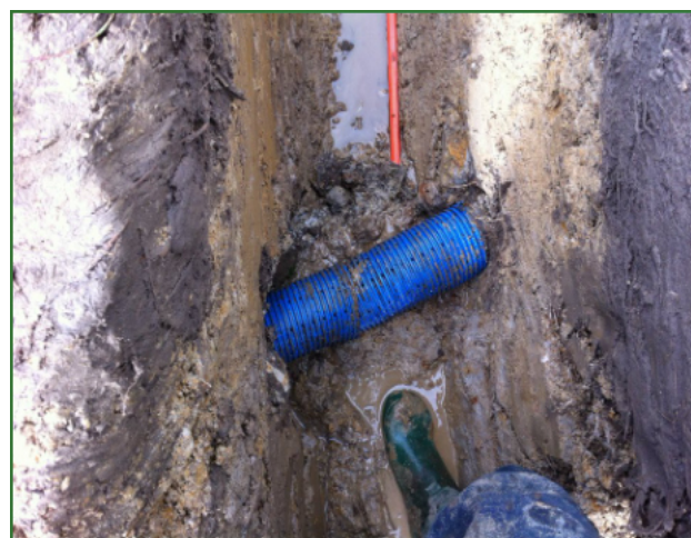
Going under septic tank drains.
