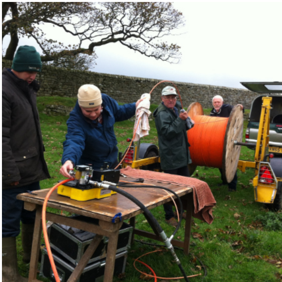
Alistair blowing the fibre over Littledale.
