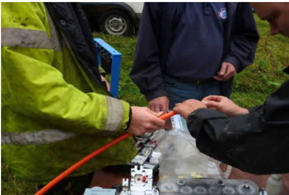
Putting the sponge into the duct.
