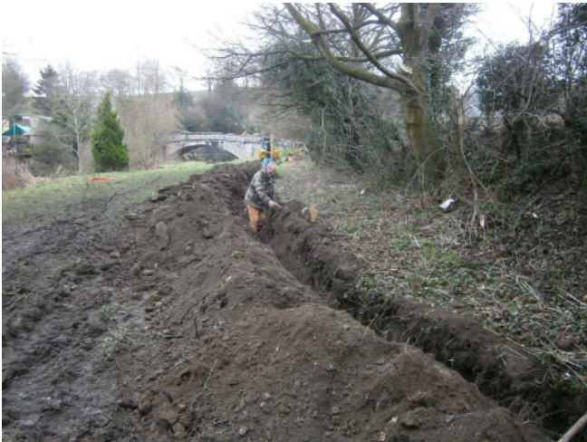
Backfilling the trench with soft fill.
