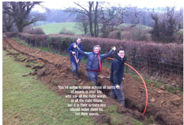
Bobbiners laying duct in the trench.
