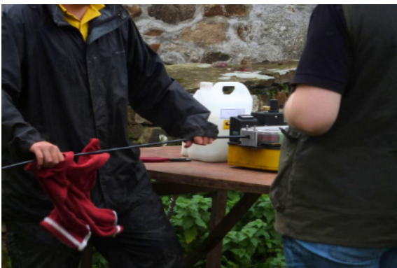
Feeding the fibre into the machine using cleaning cloths.
