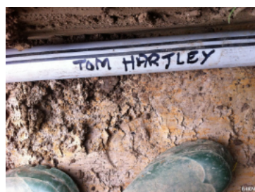
Sponsored duct carrying the fibre to the cabinet in Abbeystead
