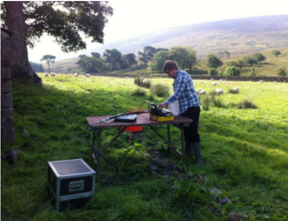
Alistair blowing fibre.
