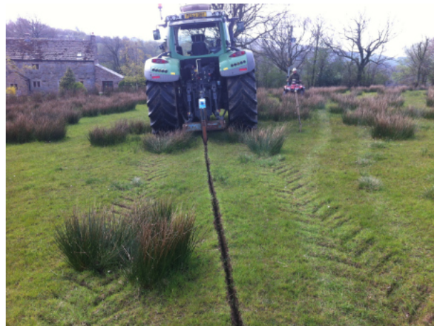
A tractor mole plough in action.
