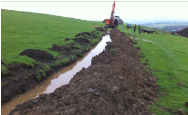
A trench dammed to run off the water.
