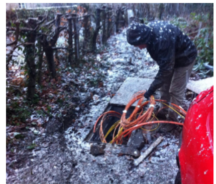
All weathers: Bruce getting customer ducts out of the chamber ready to blow fibre in.
