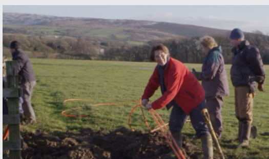
AnnaGerd putting the ducts in the trenches.
