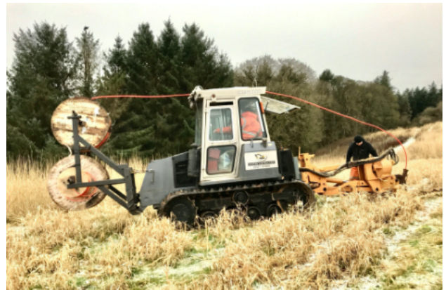
On 6th January 2022 we were ploughing in the ducting down from High Bank Hill to the Raven Beck
