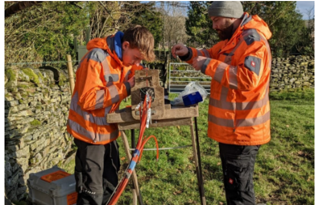
Fusing the bullets in the field chambers.
