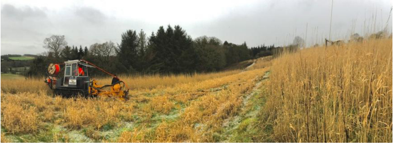
On 6th January 2022 we were ploughing in the ducting down from High Bank Hill to the Raven Beck
