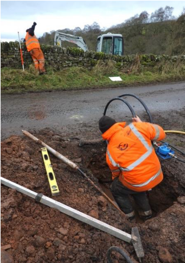
On 15 th December 2021 we moled under the road to Renwick Mill.
