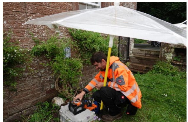
Fusing the fibre at a house.
