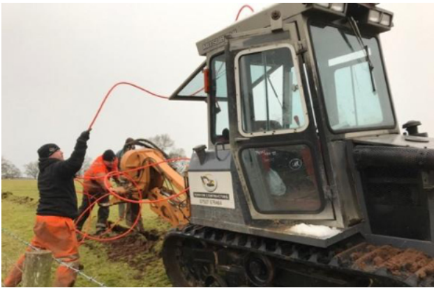
On 6th January 2022 we were ploughing in the ducting down from High Bank Hill to the Raven Beck
