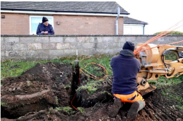
Branching off the core with a house duct.
