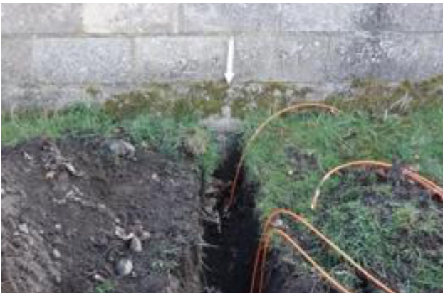
The marked spot for the house duct to enter the property.
