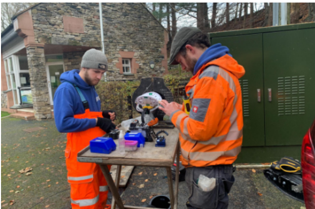
Fusing the chamber bullet to bring everything live.
