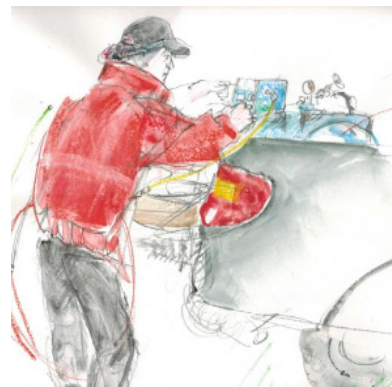
Barry using the nano to blow the fibre to Flick.
