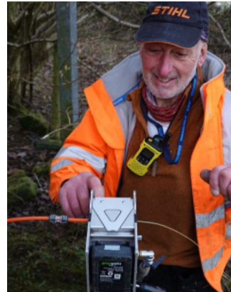
Barry using the nano to blow the fibre to Flick.
