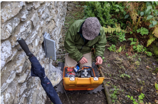
Tim fusing customer connections.
