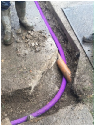
Sub-ducting when needed. Some careful work to avoid existing utilities.
