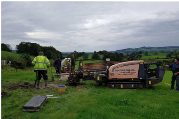
Drilling under the A6 at Stocks Mill for Route 7 - September 2020.
