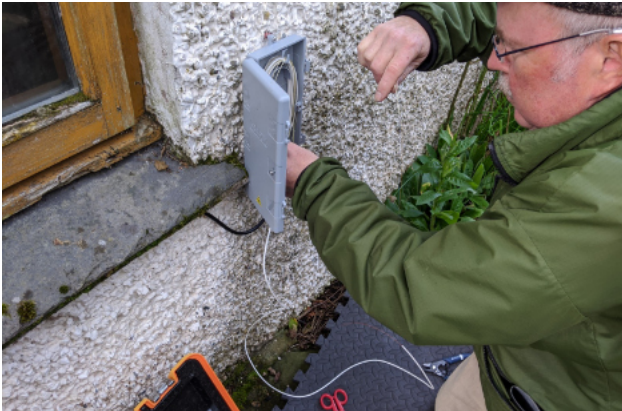
Tim wrapping the fibre in a customer connection.
