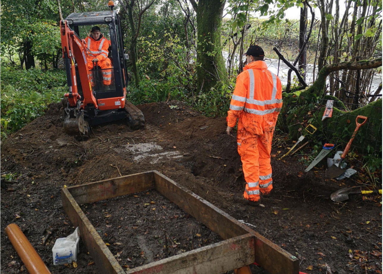
B4RN civils building the base for Grayrigg cabinet.
