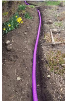
Sub-ducting when needed. Some careful work to avoid existing utilities.
