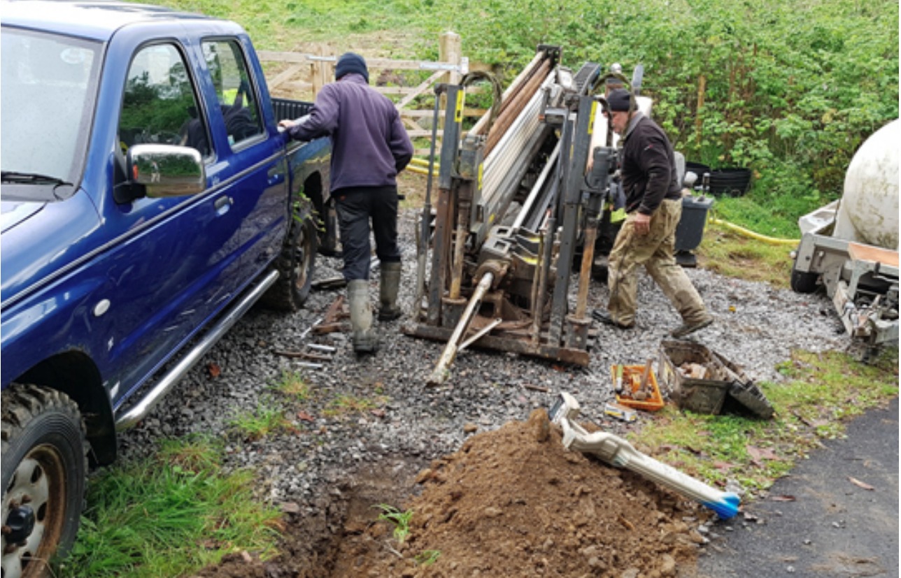
Swinny drilling under Gurnal Bridge Lane.
