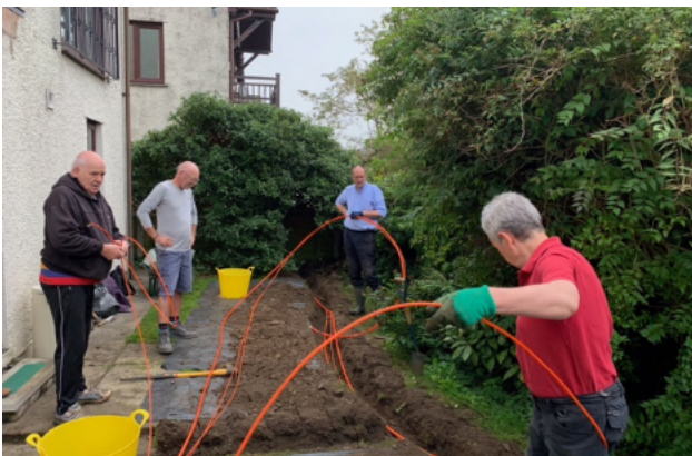
Multiple ducts in the trenches.
