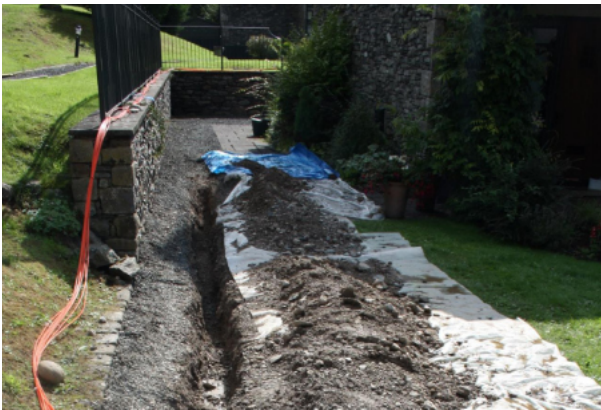
Trench ready for levelling and duct placement.
