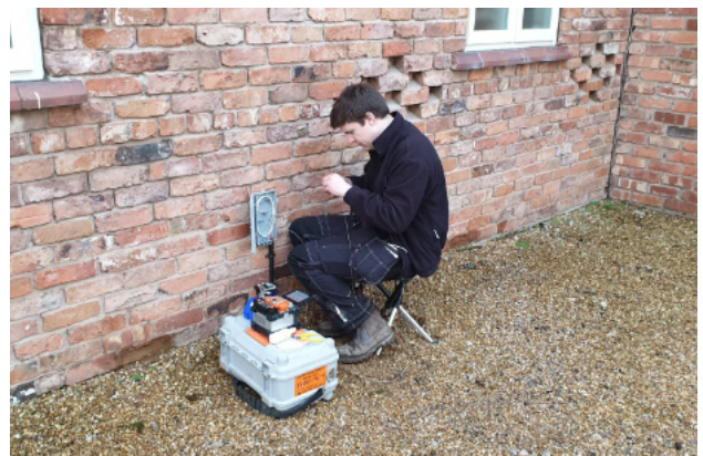
B4RN splicers fusing the house connections.
