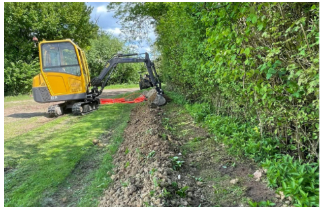
Backfilling.
