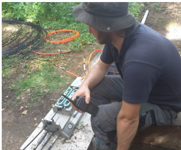
James blowing core fibre.
