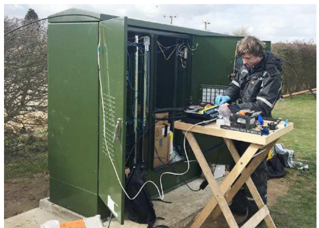
Matt Mercer fusing the fibre at the cabinet.
