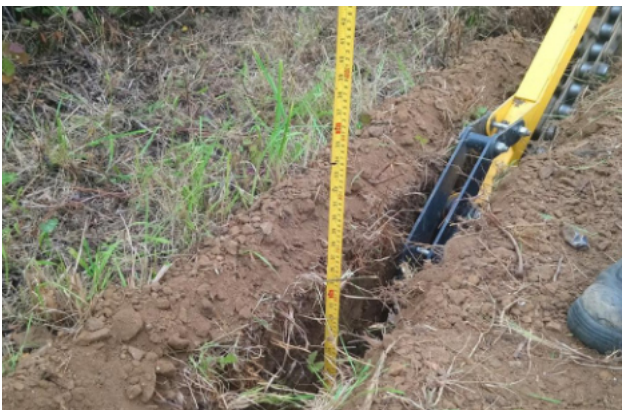
Checking the depth of the trench.
