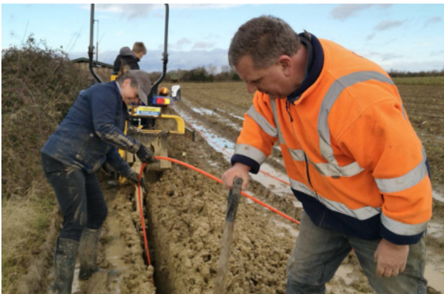
Laying the duct in the trench.
