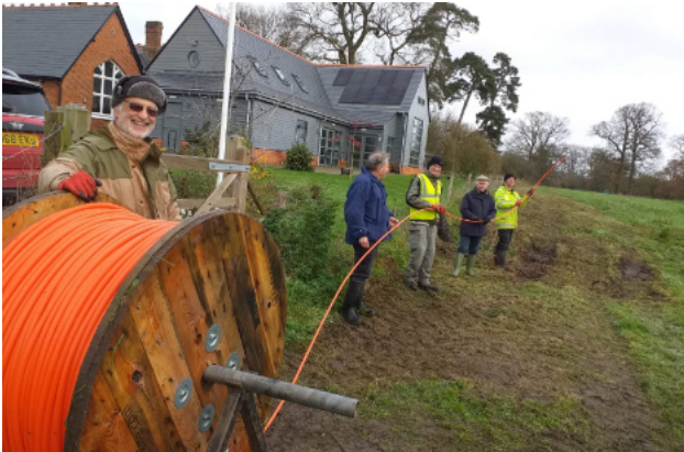
Reeling out the duct.
