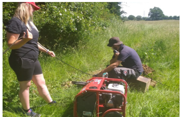
Ashley and James blowing core fibre.
