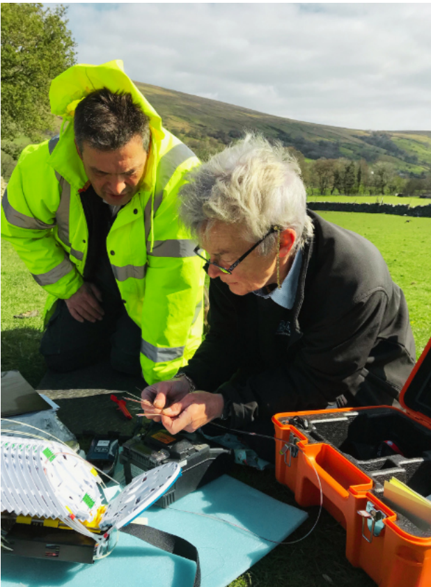
One of the northern volunteers, showing a new volunteer (David Evans from Norfolk) how to fuse fibre-optic cable in a field at Dent. David became a B4RN employee and looked after the Norfolk network. Photo by Kira Allmann.
