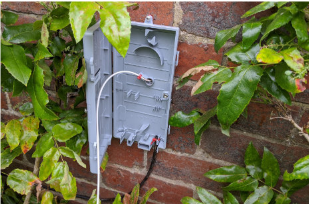
Will fitted the external house box and threaded the fibre through.
