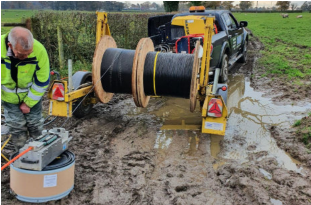
Frank Brown blowing core fibre.
