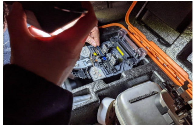
Flick putting customer fibre in the splicing machine by torchlight.
