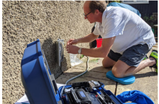
Charlie Bowman fusing connections at Whitewell.
