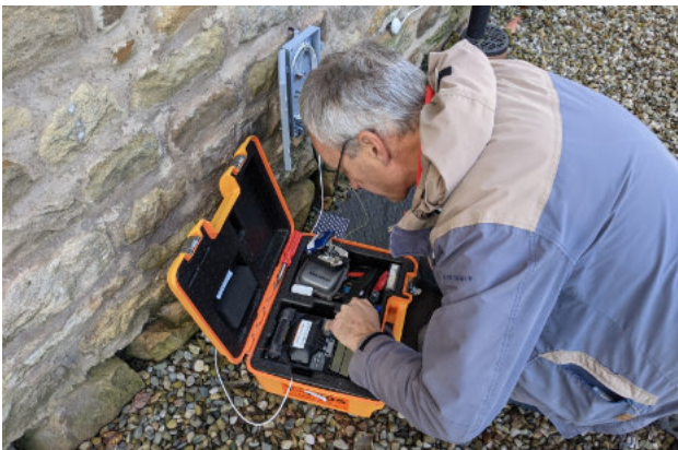
Guy Campion fusing the outdoor connection.
