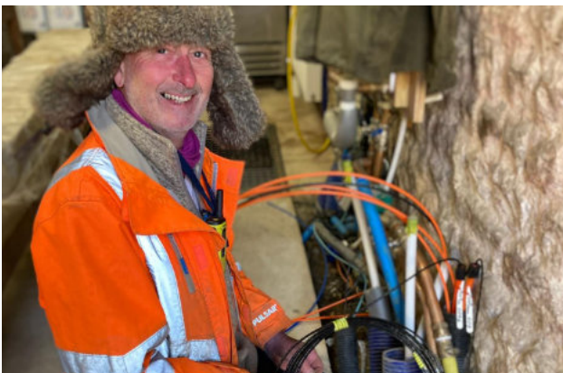
Barry from B4RN blowing fibre.
