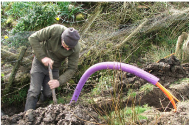
Subducting the core duct.
