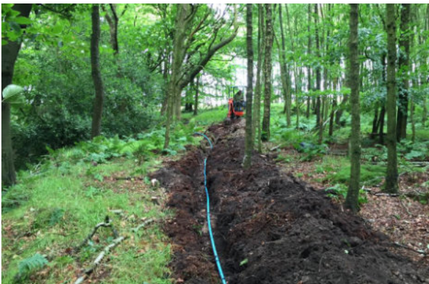
Sub-ducting (water pipe) through the woods.
