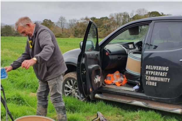
Frank blowing house fibre.
