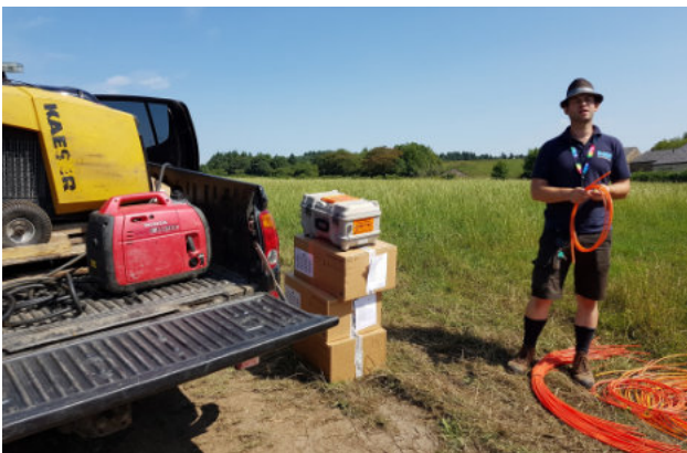
Paul Parsons blowing fibre into house fibre ducts.
