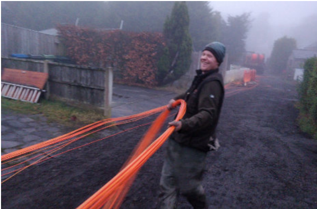
Kurt, one of Roger Clark's team, installing multiple ducts from Head End.
