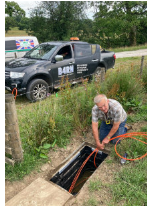
Fran Brown blowing the core duct.
