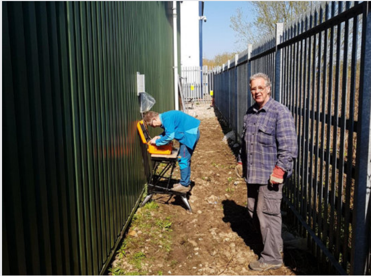
Christina fusing the customer end of the connection.
