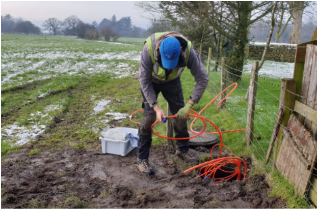
Guy connecting ducts in the small chamber.
