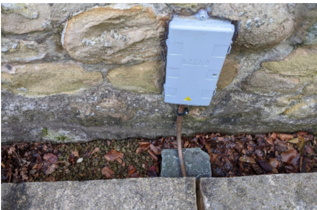
Belt and braces, duct run through spare copper pipe under the flags.
