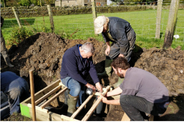
Getting the base ready for concrete.
