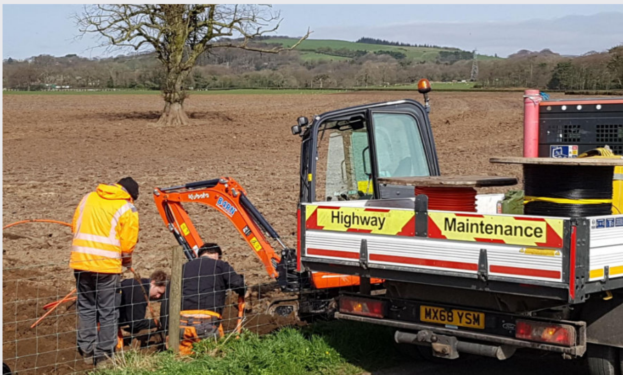
The B4RN team repairing and rerouting a severed duct.
