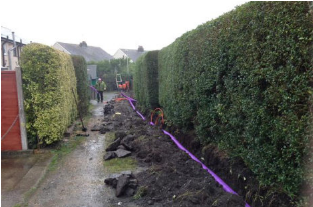
Using subduct where it could not be buried deep.
