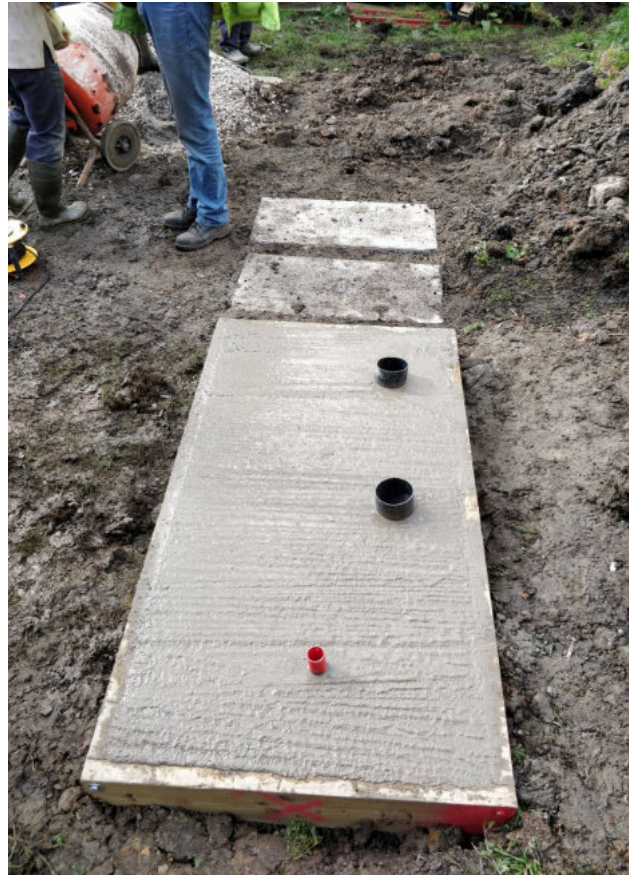
Finished plinth and chambers.
