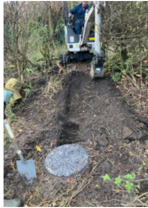
Round Chamber install.
