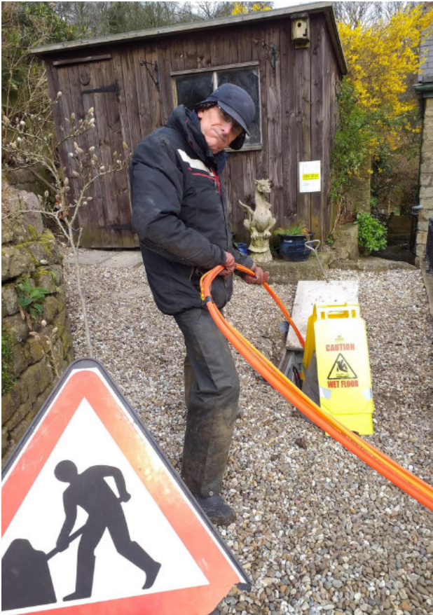
Tim Forshaw helping to install 16mm duct feeding Victoria Terrace.
