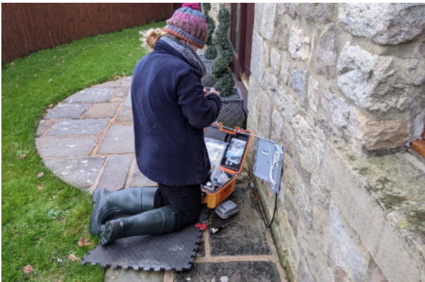
Flick fusing house connections.
