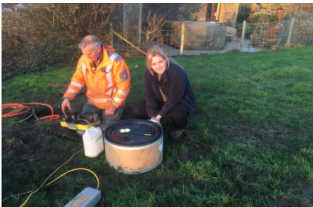
Frank and Flick blowing house fibre.
