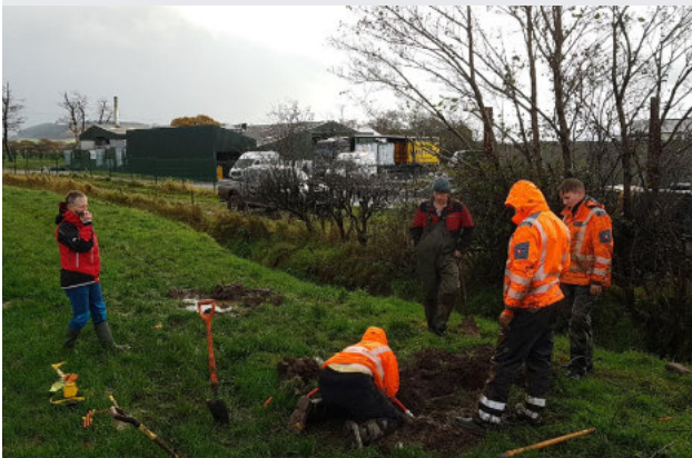
Chopping out a blocked duct on the core 288 fibre.
