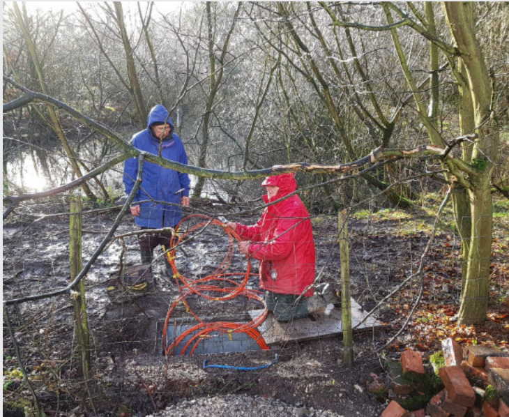
Tim and Frank blowing core fibre.
