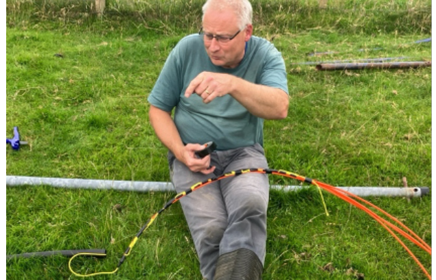
Threading duct.
