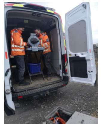
Fusing at the chamber.
