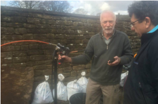
Bruce Alexander came to blow the fibre to the houses.
