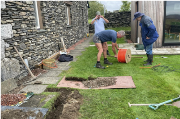
Digging the fibre to the properties.
