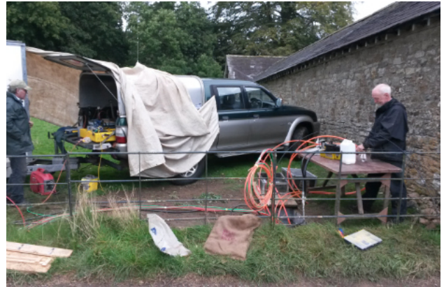
Double fibre blow at Manor Farm, of core and house fibre with Chris and Bruce..
