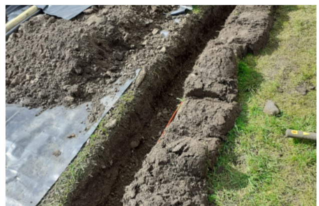
Duct in the trench ready for backfill.
