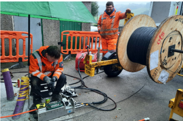
Rob Staveley and Ronan Halstead blowing core fibre.
