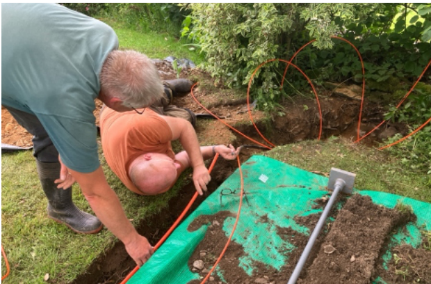
Keeping everything tidy and sub-ducting the 7mm in gash 16mm.
