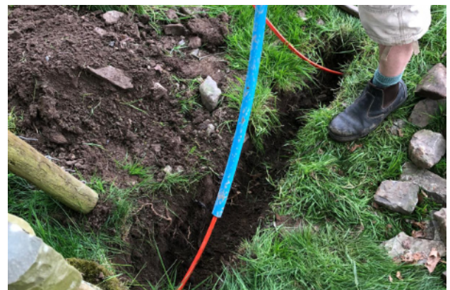
The Alkathene will protect the duct as it goes under the wall.
