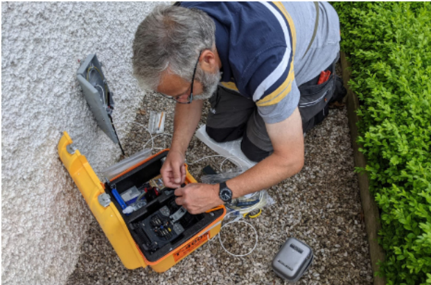
Dave fusing house connections.
