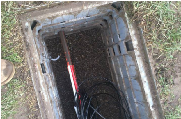
20 Metres of spare fibre blown into the chamber.
