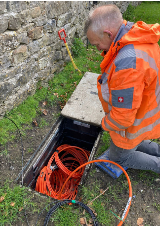
Frank sorts all the ducts and blows the house fibres.
