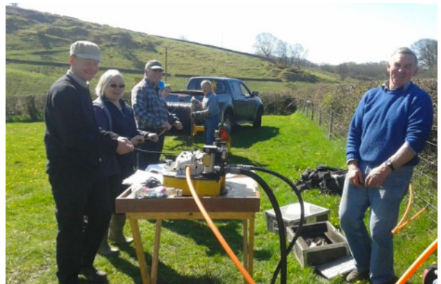
Frank and the volunteers blowing the core fibre.
