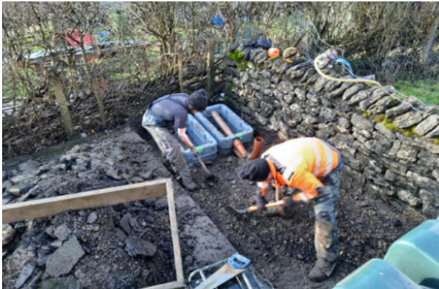
Digging out the base for the chambers and the Crosthwaite cabinet.
