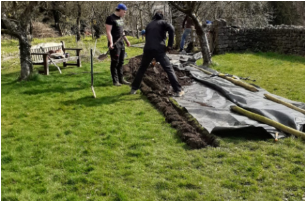
Sheets put down for spoil and sod rolled back.
