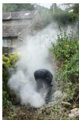
Angle grinding through rock.
