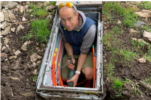
Cutting holes in a chamber.
