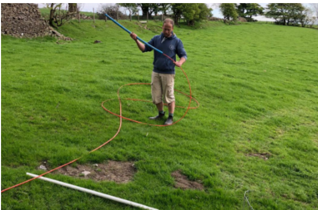
Paul threading duct through Alkathene pipe.
