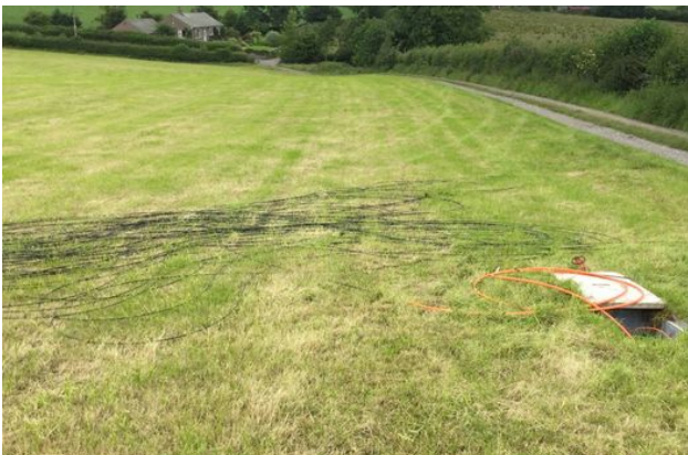
A remote fleet at a chamber on a core blow.
