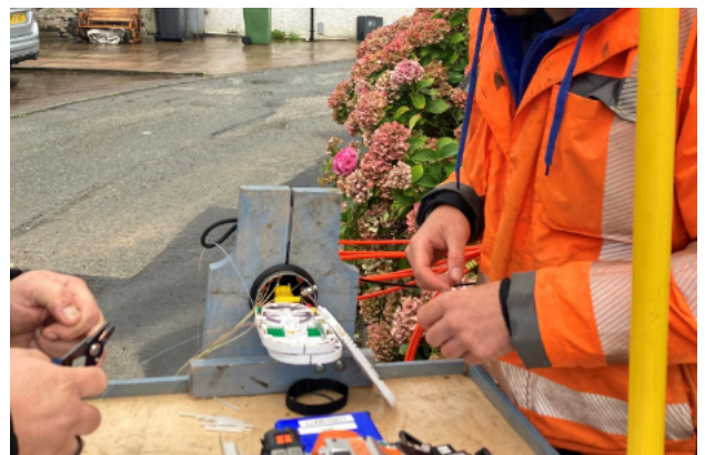
The B4RN fusers doing house connections in a bullet.
