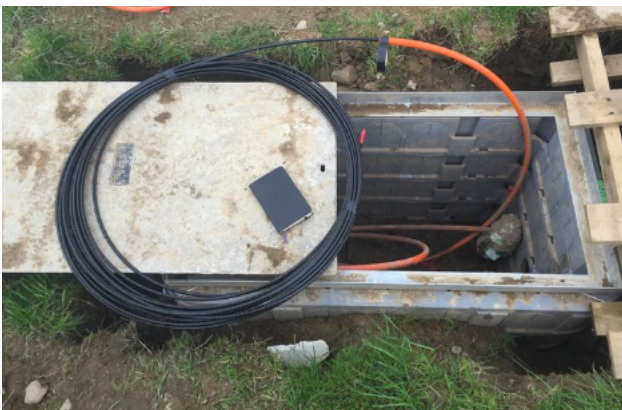
The end of the line, 20 metres in the final chamber.
