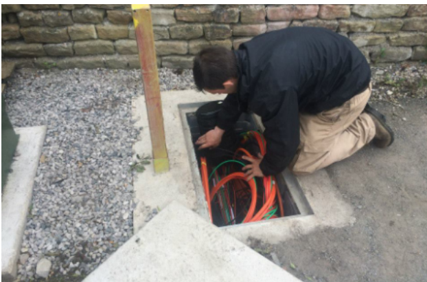
Paul puts the cabinet bullet back into the chamber.
