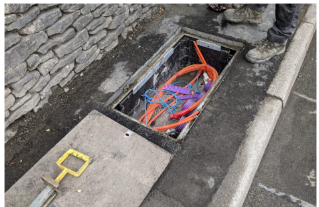
Core duct to each chamber in the pavement digs.
