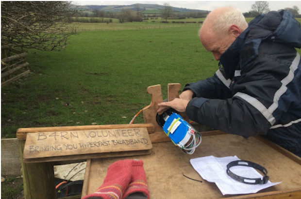
Assembling the bullet in the field.
