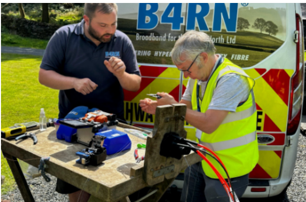
BDUK have a go at fusing the fibres in a bullet.
