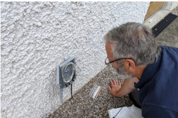
Checking the finished wrap in the wall box. No bends.
