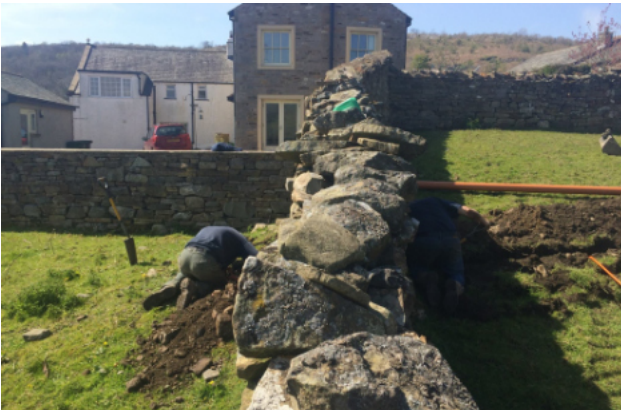
Contractors dug under the old stone walls on the core route.
