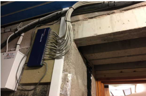
Ethernet to every room through the switch.
