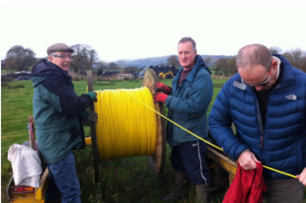
Reeling the fibre into the blowing machine.
