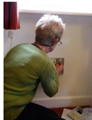
Wrapping a fused pigtail into the FTU (Fibre Transmission Unit).
