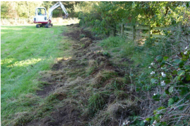
Putting the sod back on.
