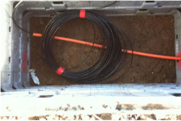
20 metres of fibre in each chamber.
