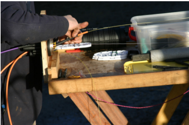
Fusing the fibre at Ivah.
