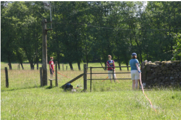
Laying duct out over the fields.
