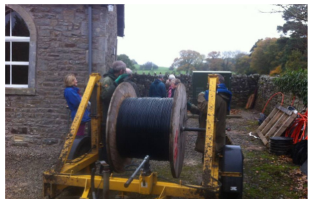
The fibre being blown from the cabinet to new routes.
