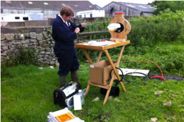
Alistair Adams-Huset fusing a bullet next to a chamber.
