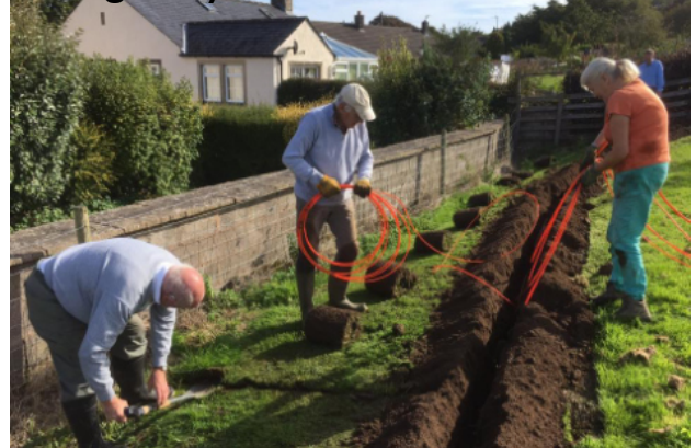
Putting the duct in the Toro trench.
