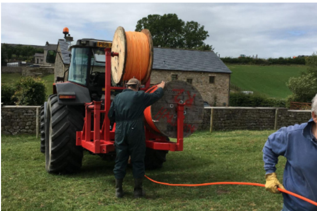
Laying the duct out.
