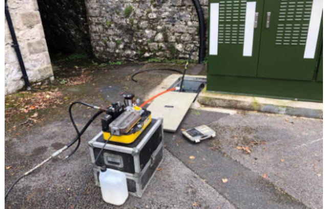
Core blowing from the cabinet.
