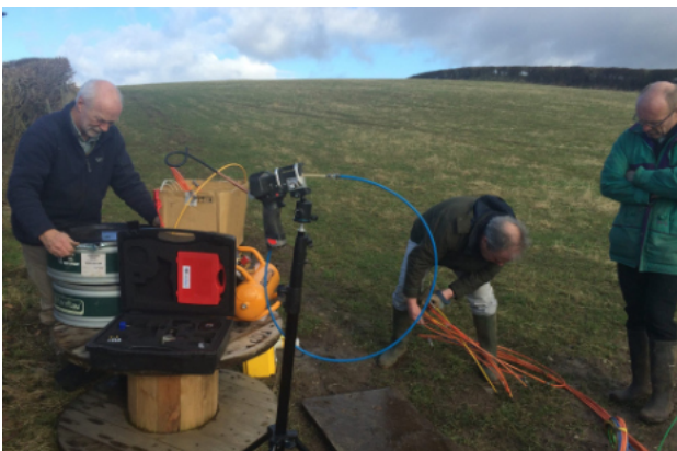
Bruce Alexander and Keith blowing house fibres at a chamber.
