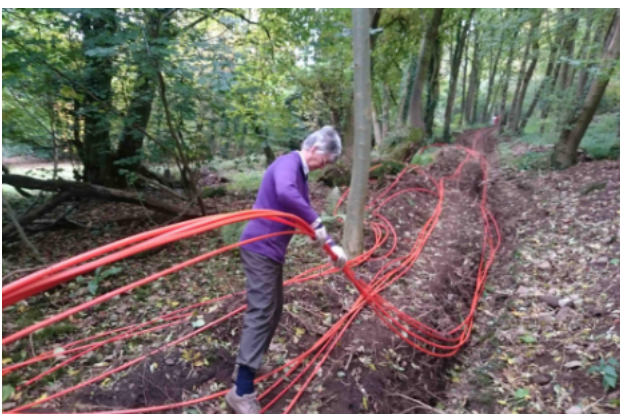
Jean taping the duct together in the Yealand woods.
