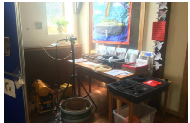
Bruce blowing fibre from the church, to the chamber.
