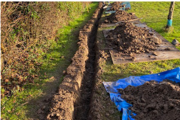
Using tarpaulin sheets keeps the grass clean.
