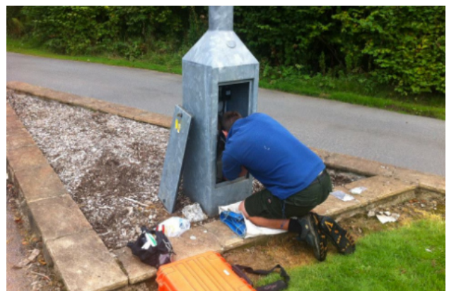
James sorting out the connection box for the cameras and wifi.
