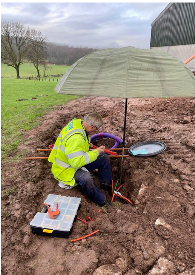
Back to reality, Martin mending a break in mud and rain.
