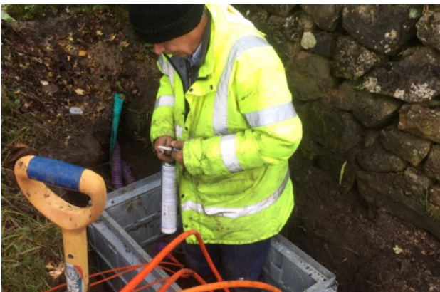
Nick Ward checking the ducts and labelling core ducts.
