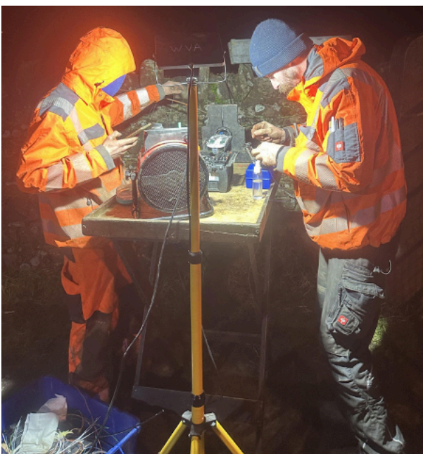
Dan and Ioan Leonti fusing one of the bullets to bring the customers live again.
