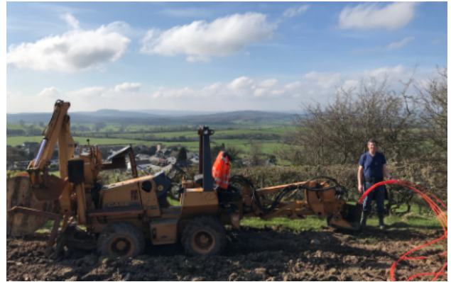
Mike helping out with the mole ploughing between Dalton and Burton to bring the core into the village.
