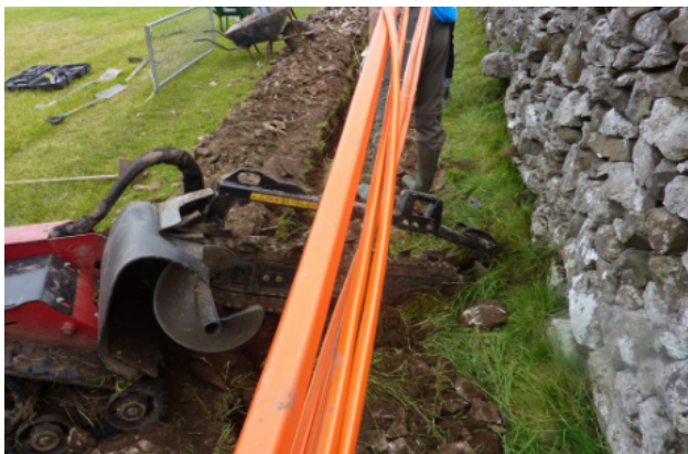
Multiple ducts being laid in the toro trench.
