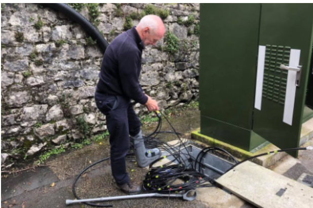
Bruce with his peg leg tidies up the core fibre in the cabinet chamber.
