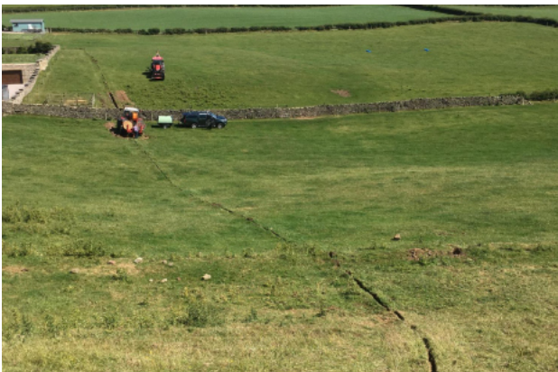
Moleing the duct and digging through gateways to the site.
