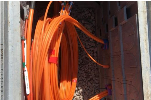
Labelled up and tidy for the blowers.
