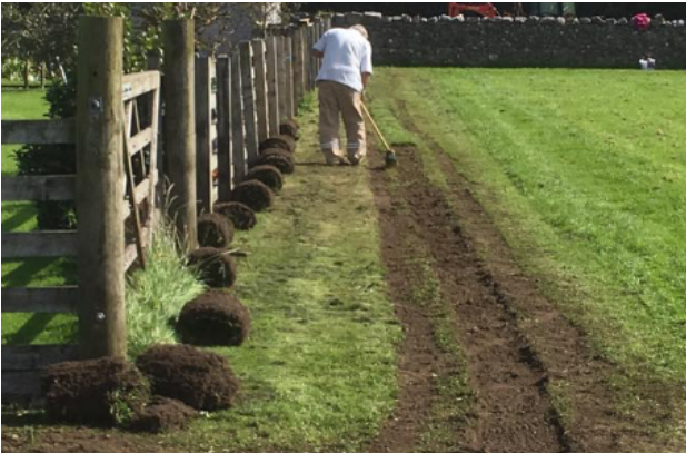
Brushing in the spoil and replacing the turf.
