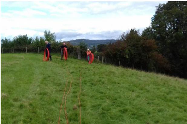
Laying the duct ready to go to the houses.
