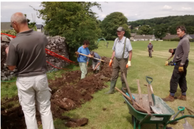
Soft backfilling the trench and removing stones.
