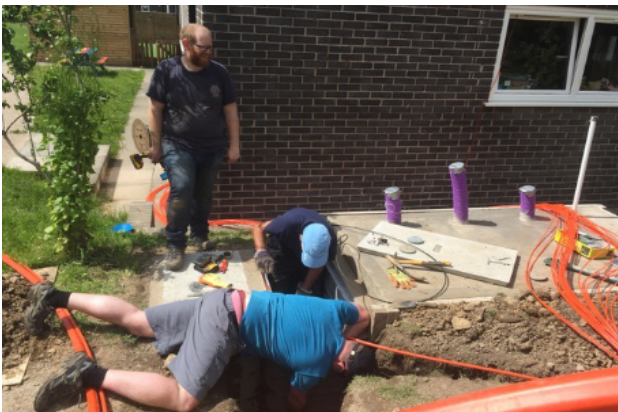
Getting the ducts through from chambers to cabinet, are Nick Martin, Sue Caddy and Ollie Craig.. Photo by Mike Iddon
