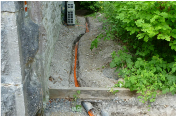
Work round the hardcore to get the house ducts to the offices.
