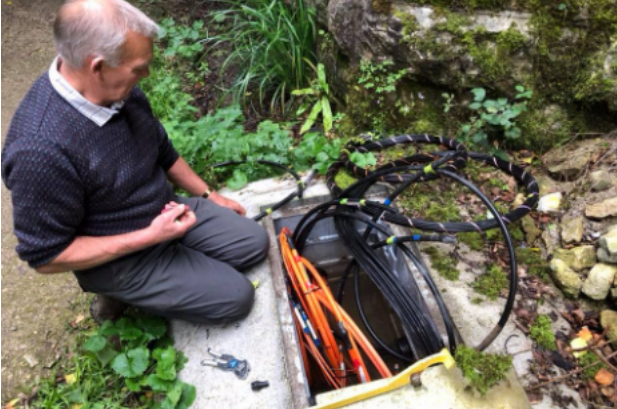
Frank Brown catching the fibre and labelling it up at the chamber.
