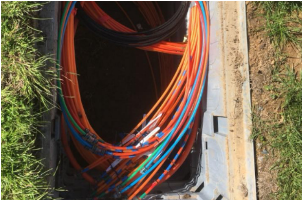
Another chamber with multicore ducts labelled up.
