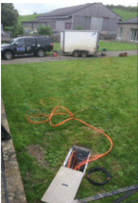
Finally the core blow to the Hall.
