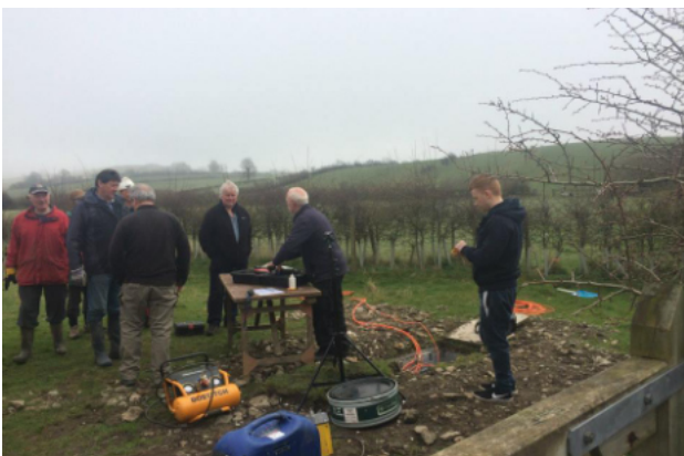
Blowing the core fibre.
