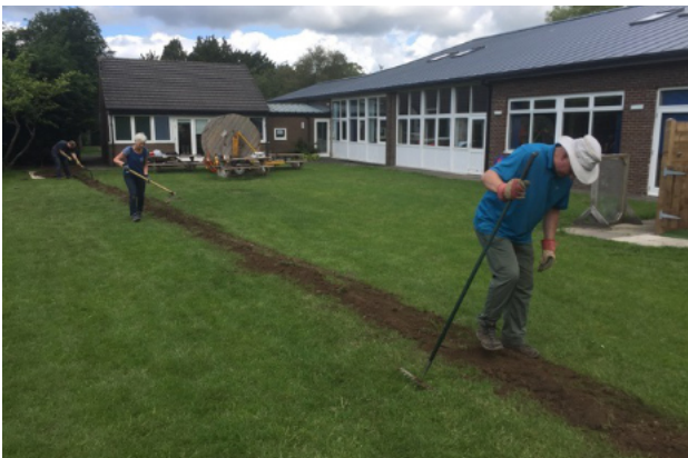
Steve Thexton backfilling the trenching the duct is in the trench.
