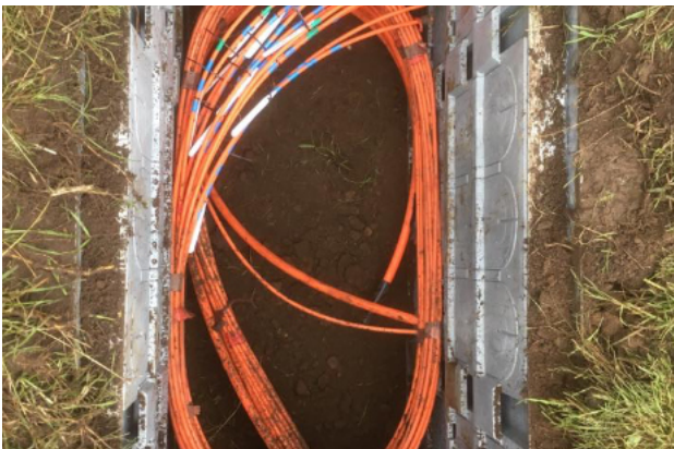
All the duct in the chamber, labelled up ready to blow.
