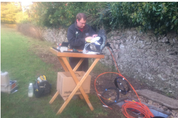
Alistair Adams-Huset fusing the core fibre at Silverdale.
