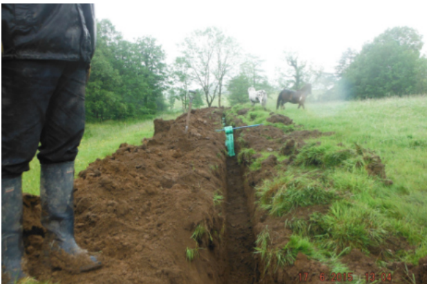
Neat trench, soft filled and tape going under the sod.
