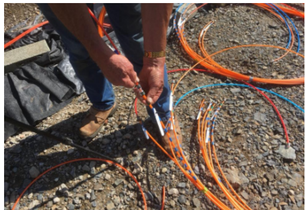
Frank puts a blowing tail on the duct he’s going to blow next.
