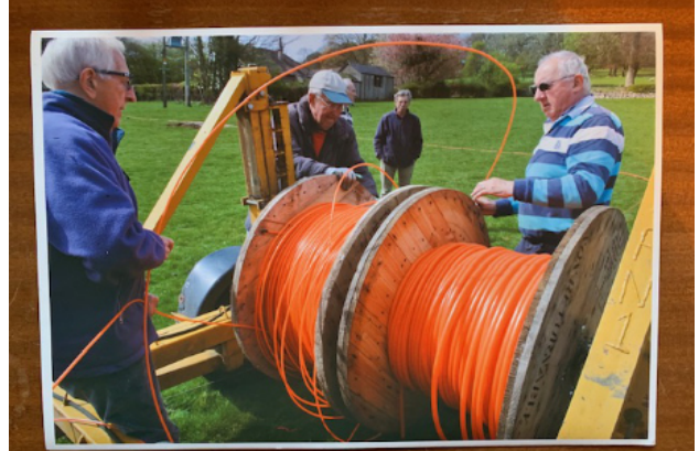
Reeling out the duct.
