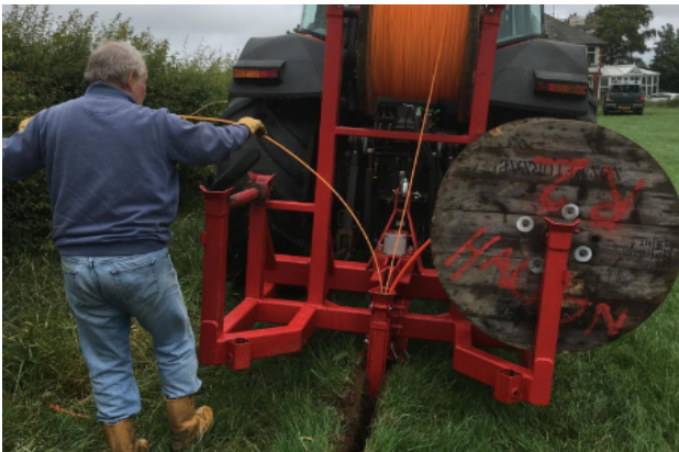
Feeding the duct into the mole.
