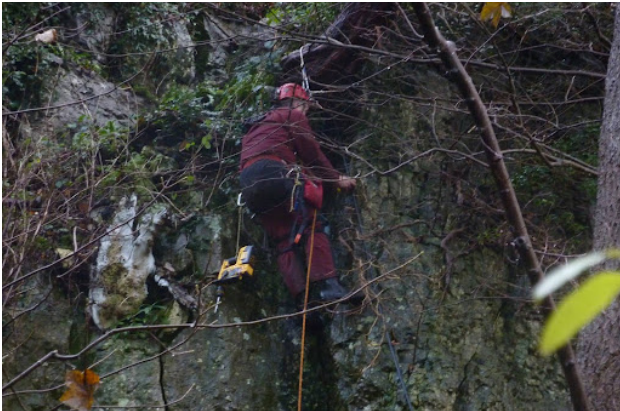
Dave Ryall from B4RN fixes external duct to solid rock.
