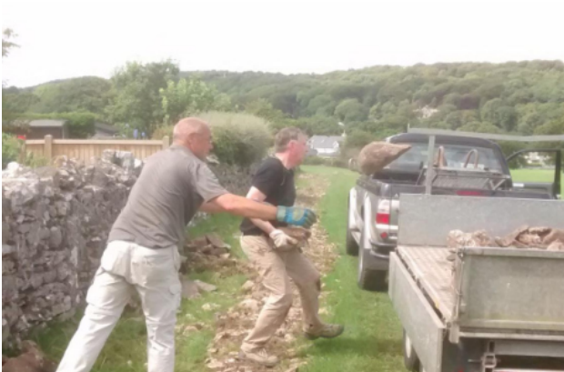
Clearing the trench of surplus stones.
