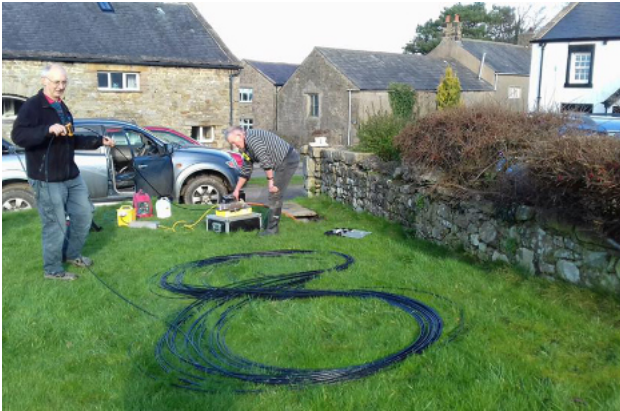
Will Dehany un-fleeting core fibre as Frank blows it to the next chamber.
