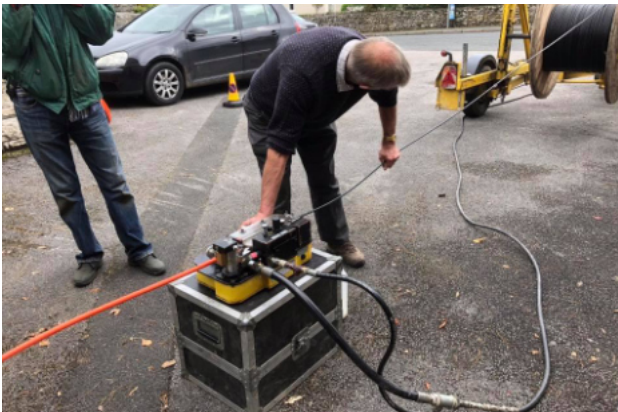
Frank on the core blow machine.
