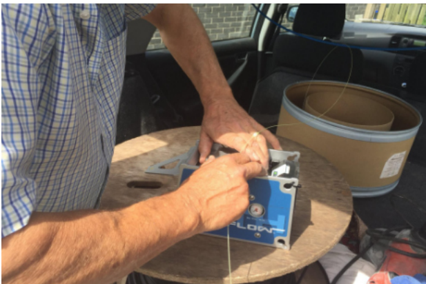
Martin Lange blowing the fibre into the school.
