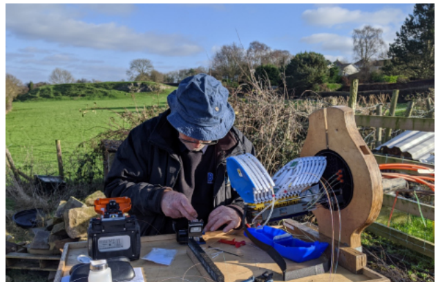
Bruce Alexander fusing the house fibre into the bullet from the chamber.
