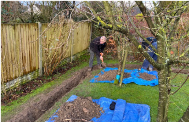
A tidy dig, with sod 'hinged'.
