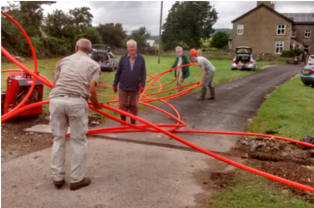
Getting control of multiple ducts.
