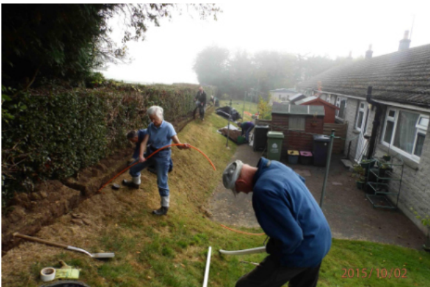
Laying ducts to the houses.
