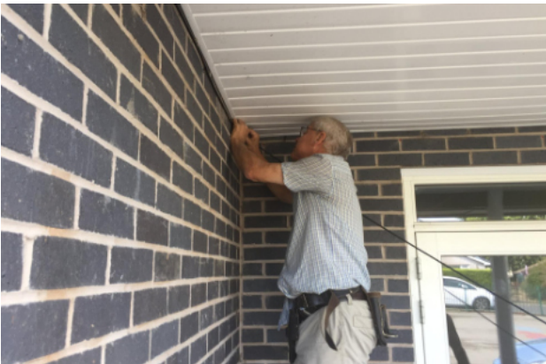
Martin Lange installing the exterior conduit on the school.
