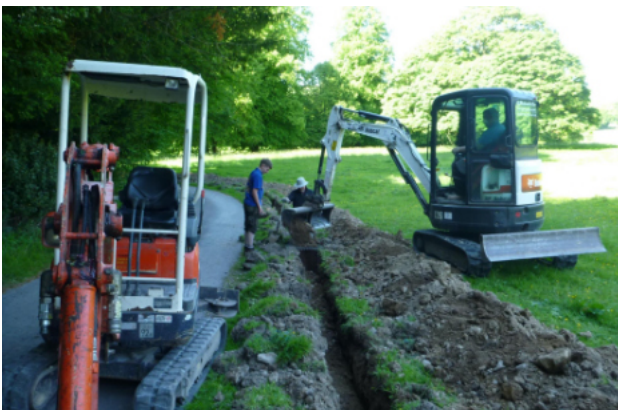
Digging and backfilling up to the hall.
