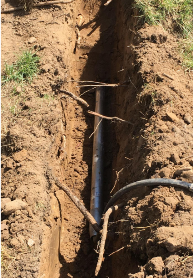
Protective pipes for subduct on directional mole.
