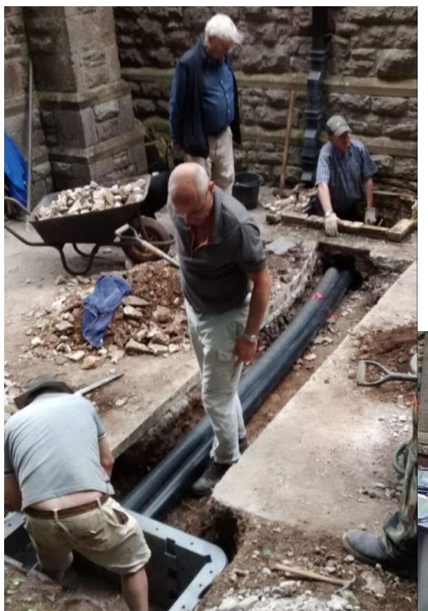
Sub-duct being laid in the trench.
