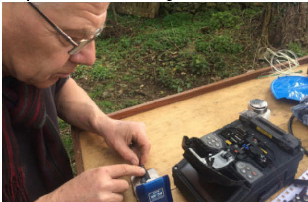
Martin fusing customer fibres in the fields.
