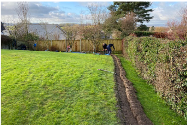
Neat hinging of the sod means the grass carries on being green.
