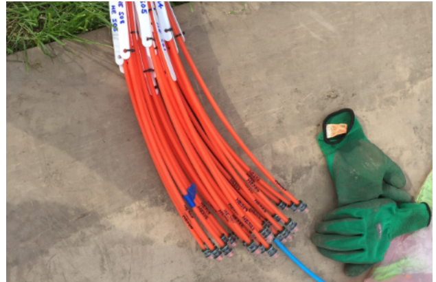
Multiple customer ducts marked up with addresses.
