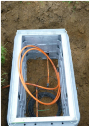
Chamber with core duct.
