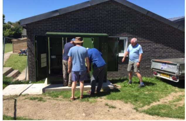
The cabinet is placed on the plinth and screwed down.
