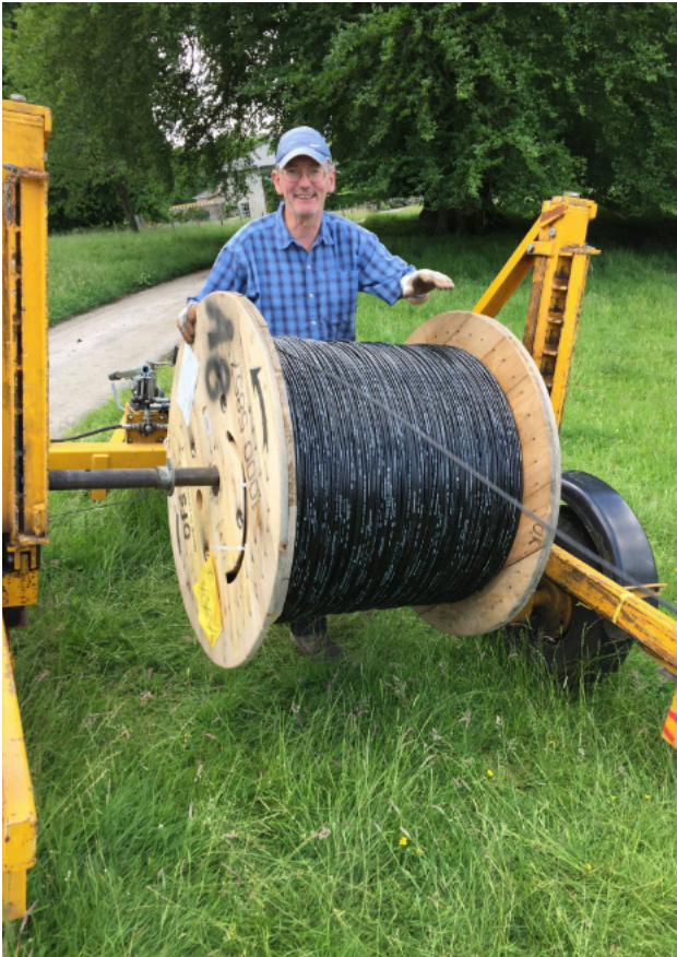
Andy reeling the core duct.
