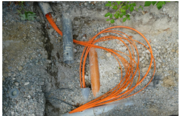
Under obstacles go the 7mm house ducts.
