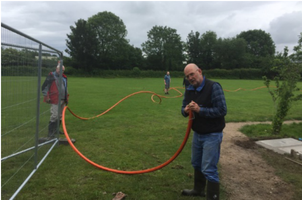
Laying the duct on the school field. Photo by Mike Iddon.
