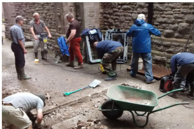
Main trench cut through the concrete.
