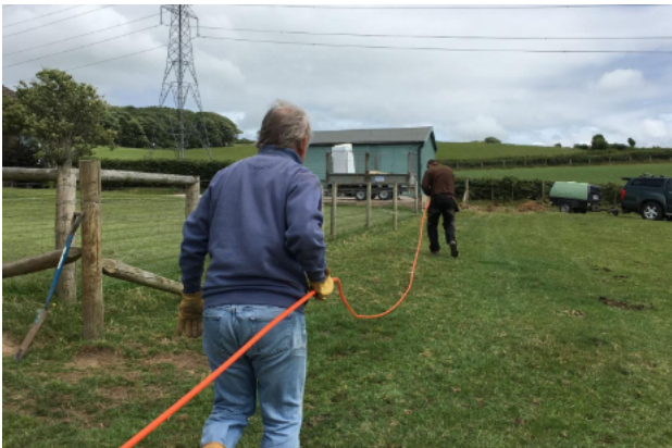
Laying duct to the caravan site.
