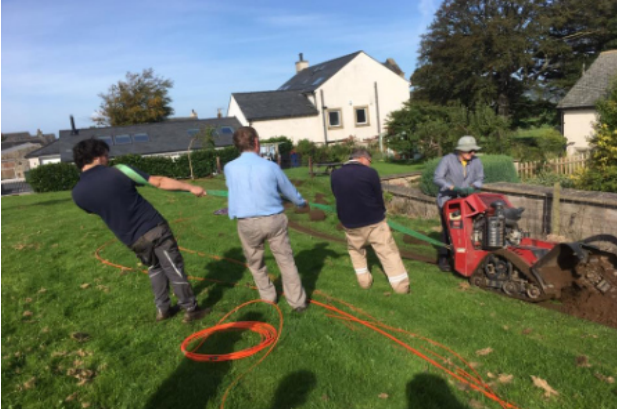
Toro, driven by Iain, with house ducts splitting off to each property.
