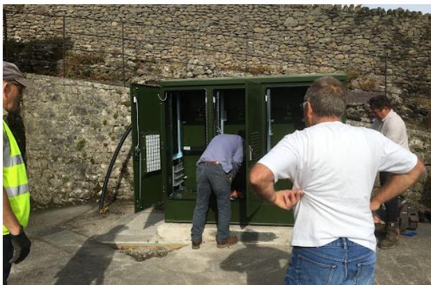
Getting the cabinet settled and ducts put through.
