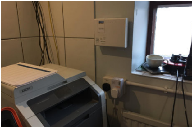
Finished installation with the router on the backplate.
