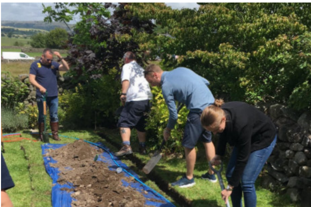
Step 2, dig out trench and place spoil on the groundsheet.
