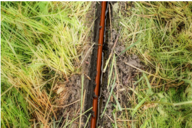
The duct in the bottom of the mole trench.
