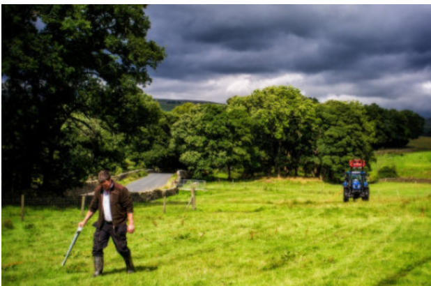
CAT scanning for utilities before digging.
