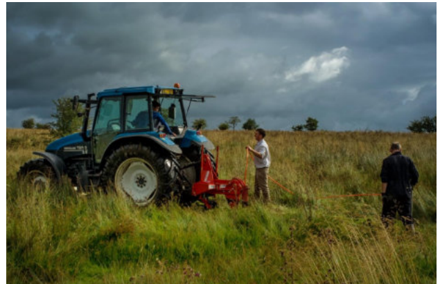
Moleing in the duct.
