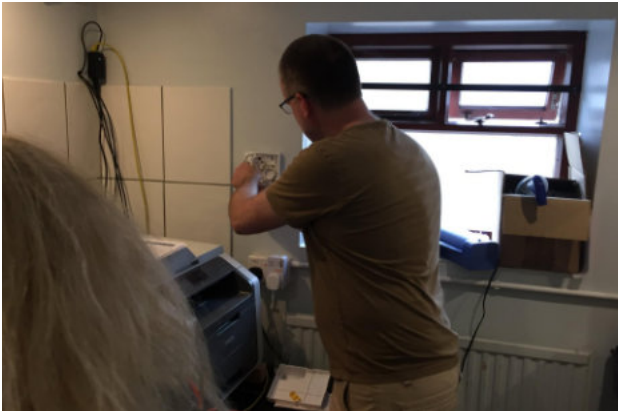
Roger wrapping the fused fibre into the backplate.
