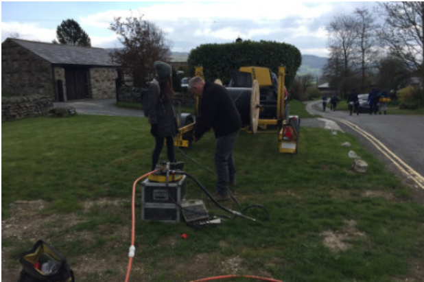
Kira watching Frank blow fibre to Will Dehany, way up the hill.
