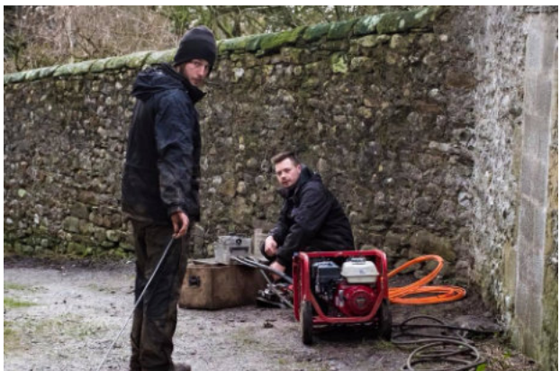
James Taylor and Sam Brown blowing fibre to Clapham cabinet.
