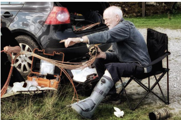
Bruce fusing customer connections into a bullet, despite his bad leg.
