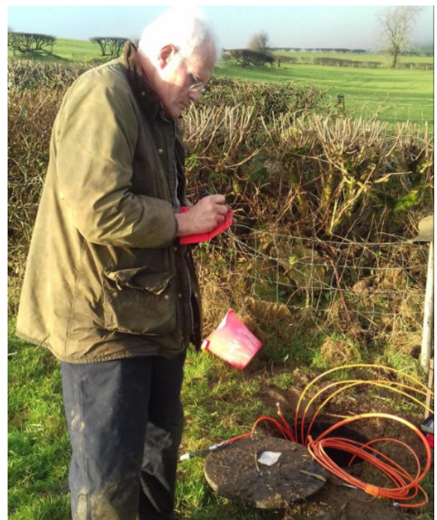
John sorting out the ducts and labelling them.
