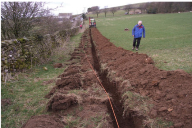
Simon laying duct in the trench.
