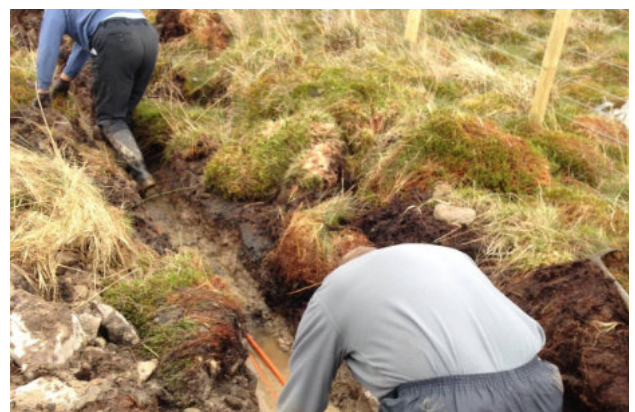
Laying duct in a very wet trench.
