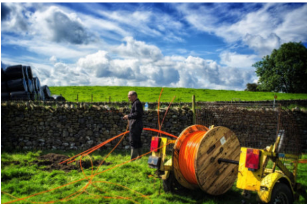
Simon reeling out duct for the trenches
