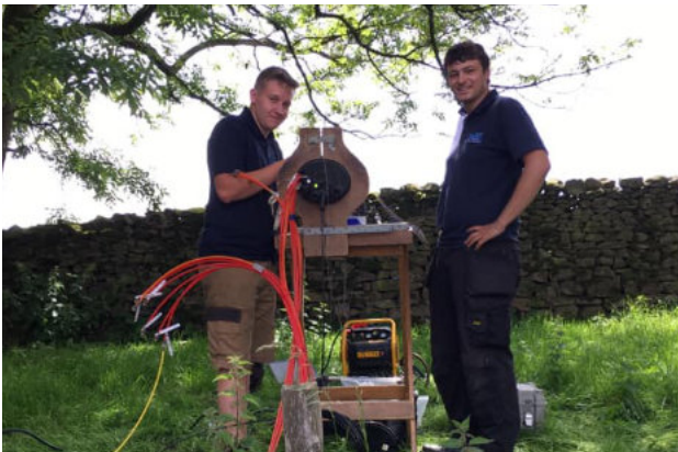
Rob and Kit fusing another bullet to bring the cabinet live.
