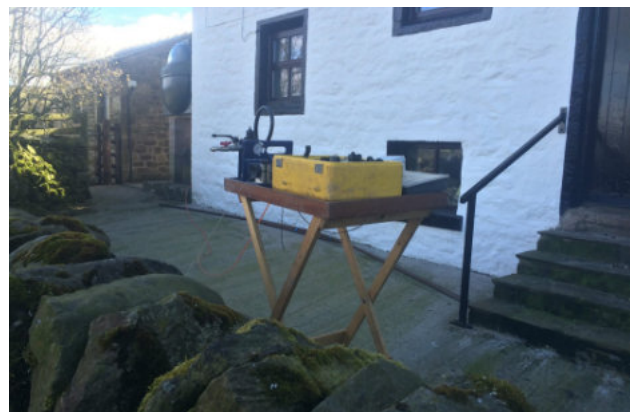
The fibre being blown from house, down to the intermediate chamber.
