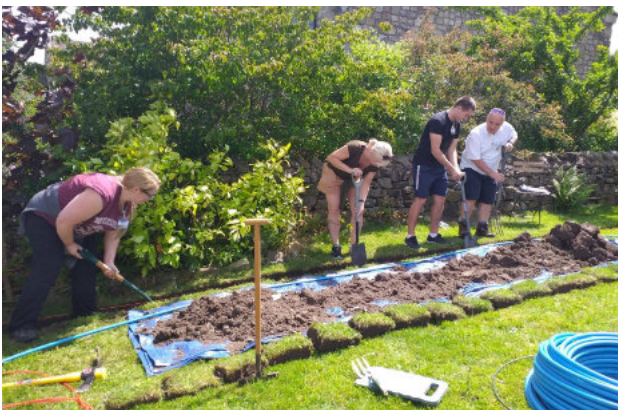
Step 3. The BDUK team having a go at trenching a garden with alkathene.
