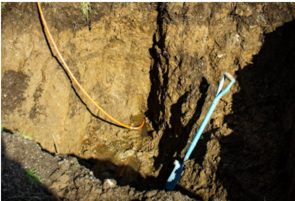
The duct threaded into the old water pipe.
