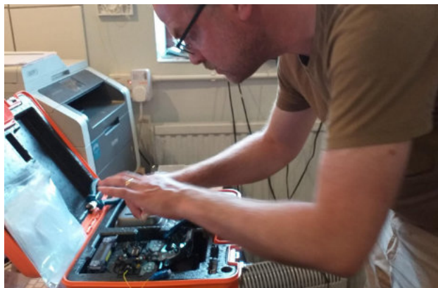
Roger fusing the house fibre in the pub.
