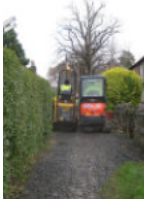
B4RN civils team duct laying in pavements and ginnels.
