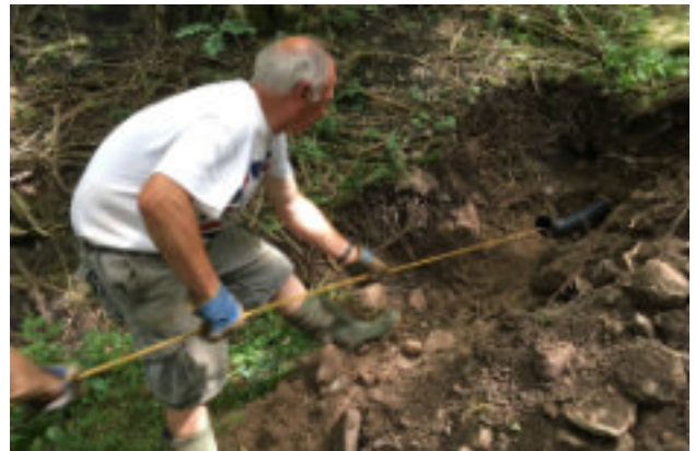
Will with the cobra getting through a duct.
