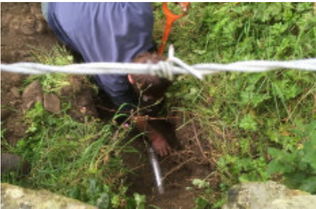
Liam from TS Trenching with the mole to go under walls and lanes.
