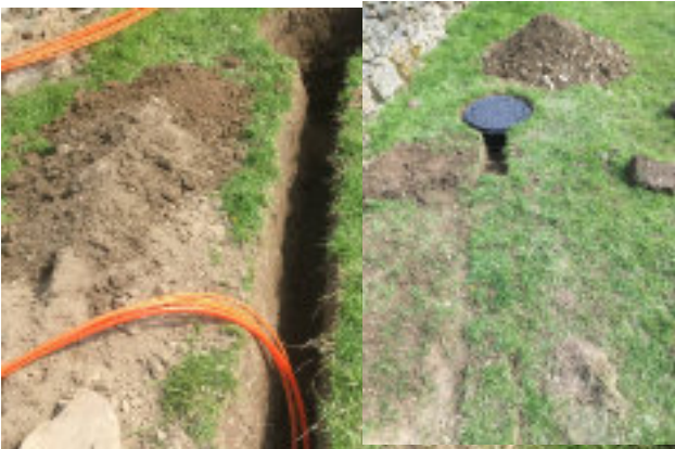
A very neat dig to a chamber and the reinstatement.
