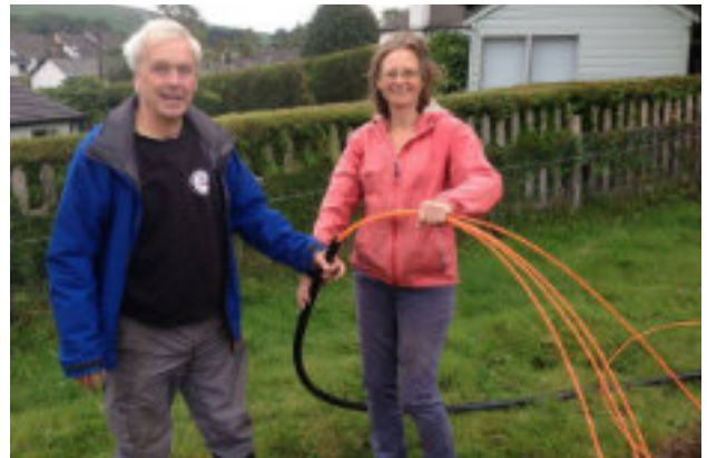
Martin Coombes and Laura Mawdsley threading four 7mm ducts down a 32mm pipe.
