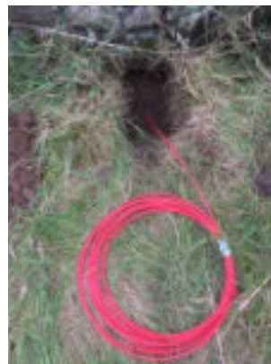
Sub ducted under a wall.
