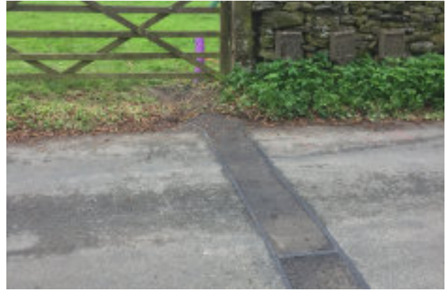
Road crossing ready to join the core dig with subduct.
