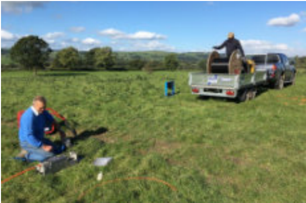
Frank Brown and Bruce blowing core fibre.
