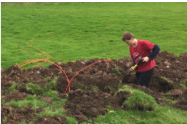
William levelling the bottom of the trench.
