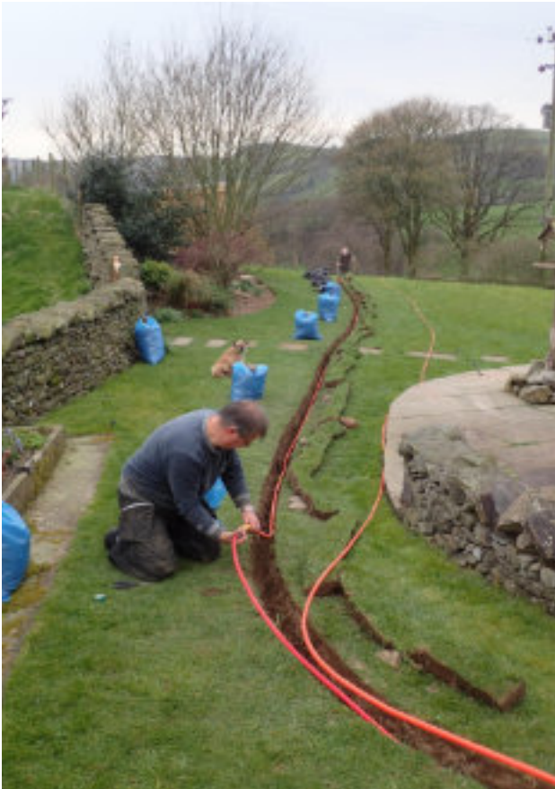
Placing the duct in the trench and back-filling.
