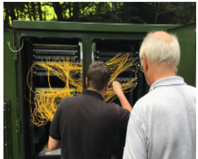
Will showing a new employee, James Clapham, how to patch in the new cabinet at Firbank.
