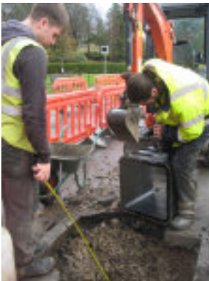
B4RN civils team duct laying in pavements and ginnels.
