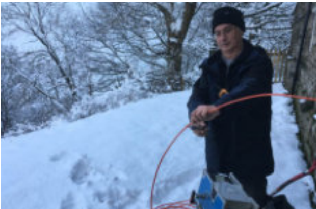
Will Dehany blowing house fibre for Gina.
