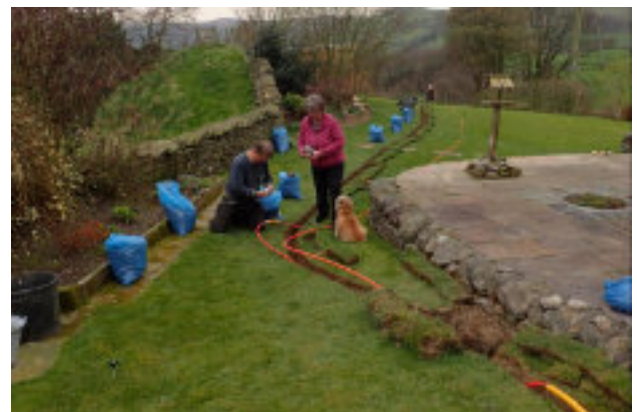
Digging the house ducts through the garden.
