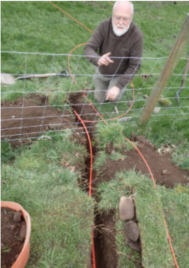
Getting the duct under the fence from the field dig.
