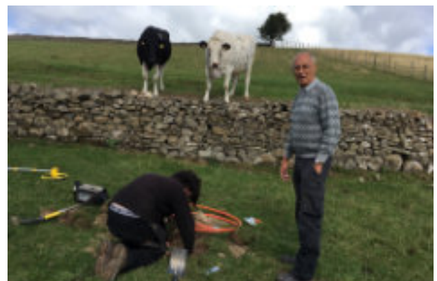
James Taylor and Will Dehany sorting out a blockage in a duct.
