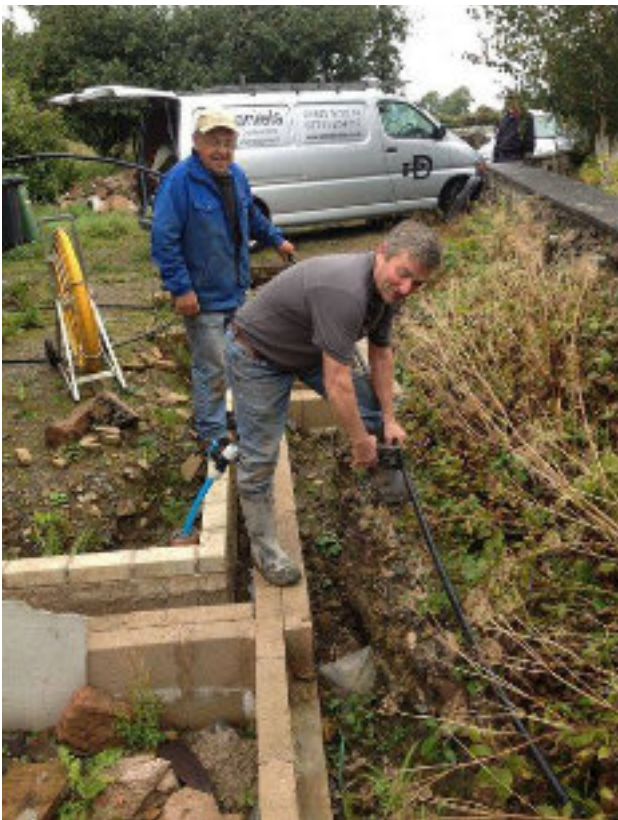
Pete Daniels prepares a protective alkathene pipe (helped by the indefatigable Raymond Gott).
