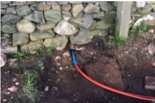
Alkathene used for extra protection.
