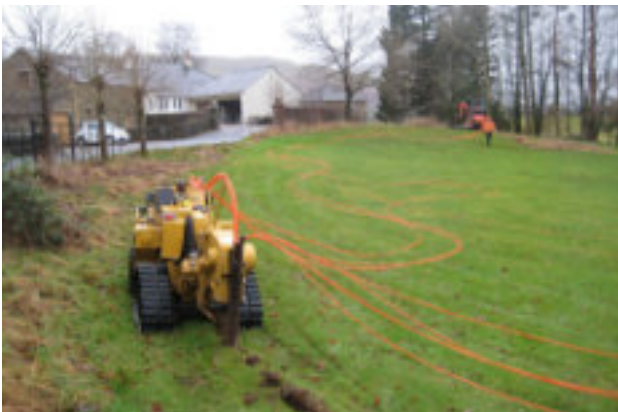
B4RN's remote-controlled mole plough at work in Douglas's wildflower meadow.
