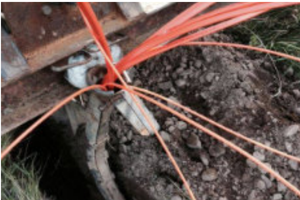
Multiple ducts in the mole plough.
