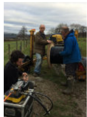
James Will and Frank blowing core fibre.
