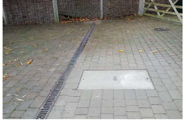
The chamber finished.
