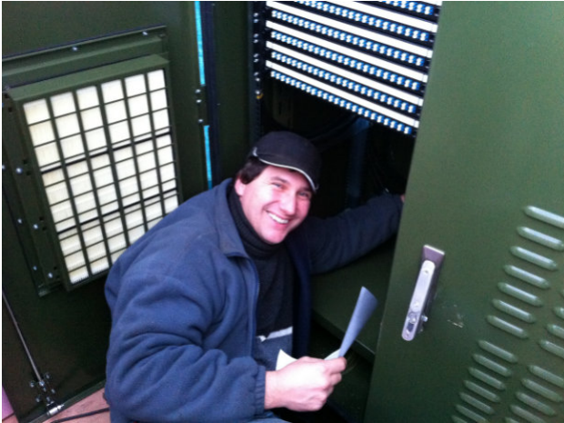
Frank fitting out the cabinet.
