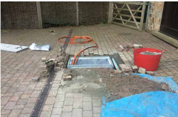
Chamber and ducts in.
