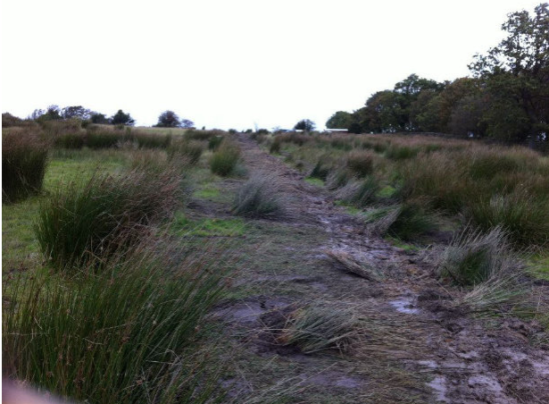
Trench through bogland with added drain.
