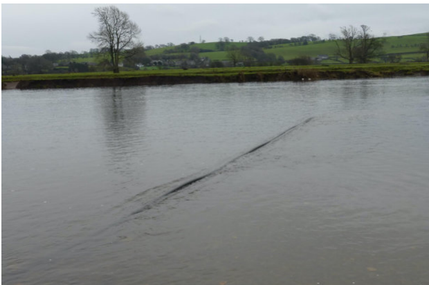
Floating duct on the River Lune.
