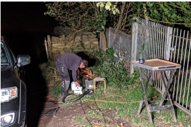
James re-blowing new fibre.
