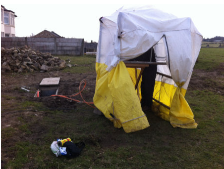
Scaffolding tent, version 1.
