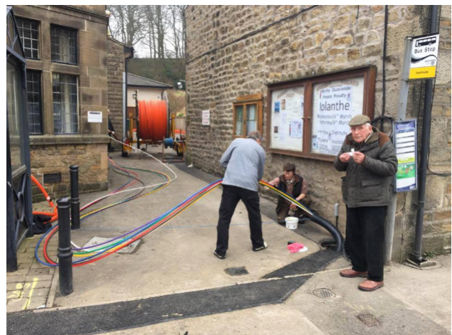
Volunteers organising the ducts.
