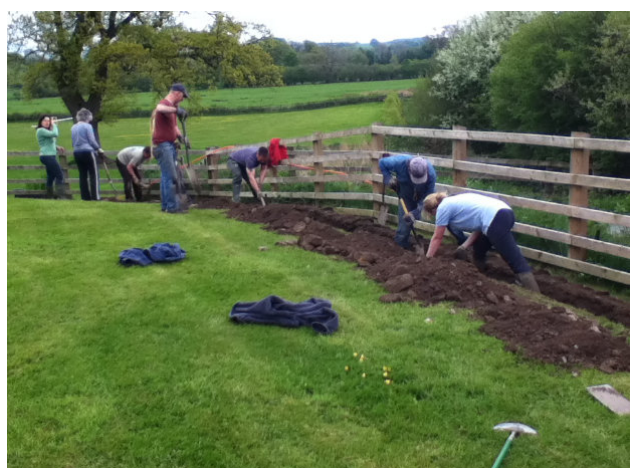
Backfilling the trench.
