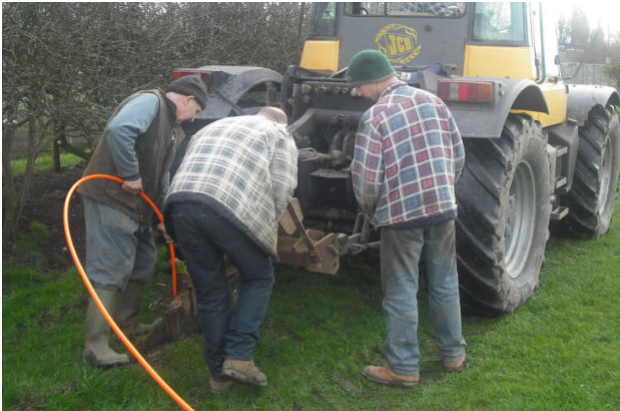
Feeding the duct into the mole plough.
