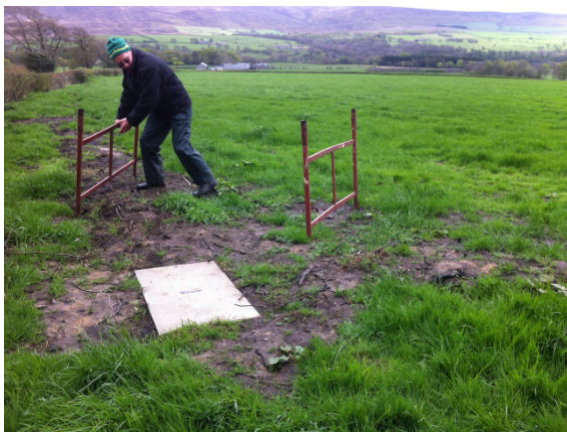
Iain building the scaffold tent.
