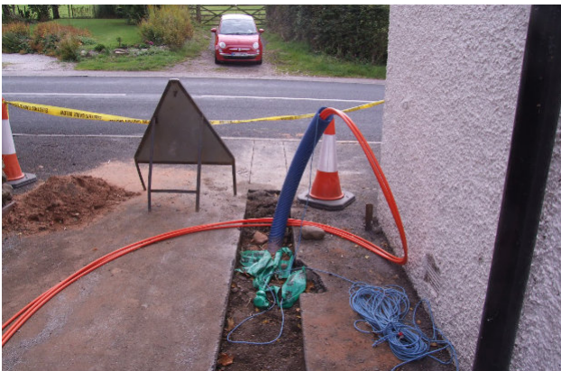
Ready for the road crossing.
