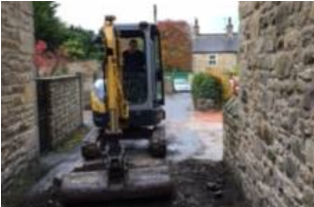
Digging down the lane to the houses.
