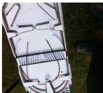
A tray with the 24 fibres ready to fuse.
