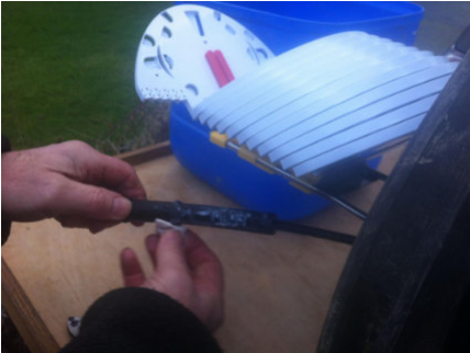
Lubricating the grommet that holds the fibres/duct.
