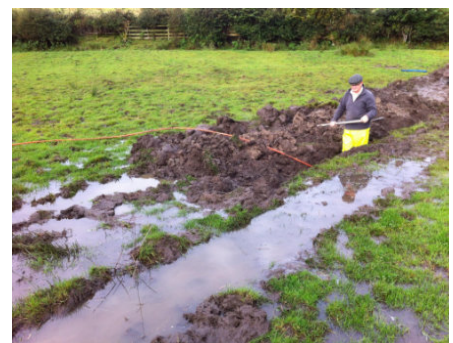
Brian Acott levelling a very wet trench.
