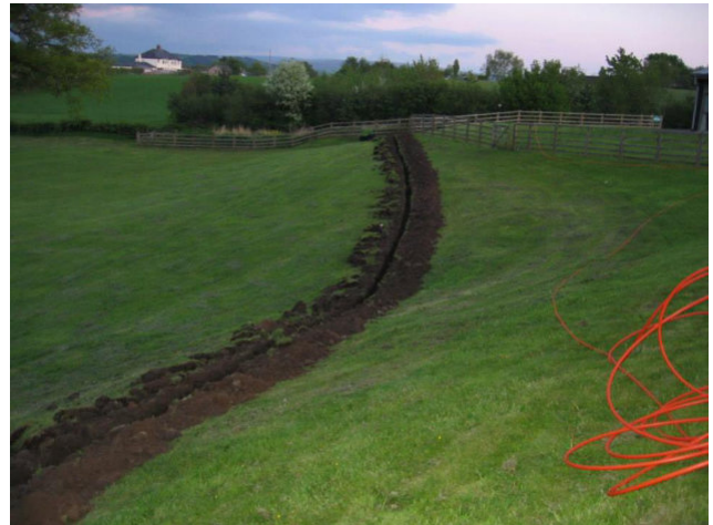
The dig down the school field.
