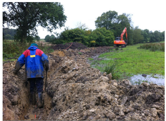
Steve Duxbury levelling the mud trench.
