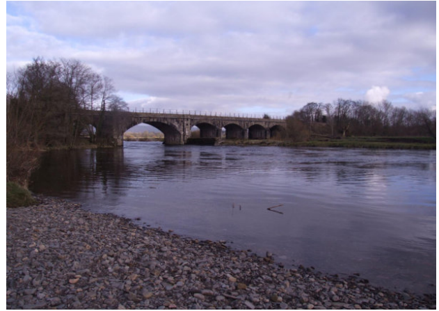
Arkholme railway bridge.
