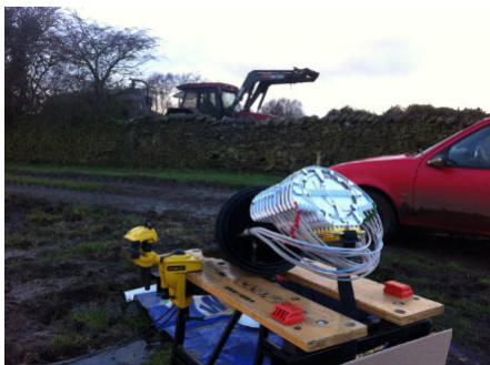
Clear tubes take the 12 fibres into the trays.
