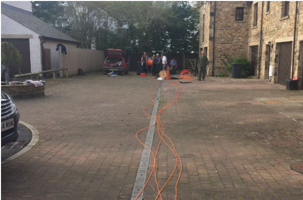
Laying out the new ducts.
