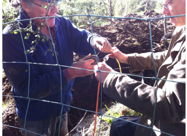
Chris Hall and Eric Lange making a join in customer duct on a long dig.
