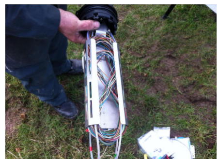
The tubes not split are coiled below.
