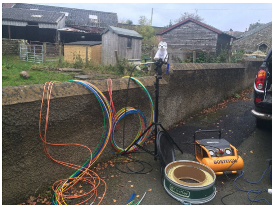
The customer tubes getting their fibre blown.
