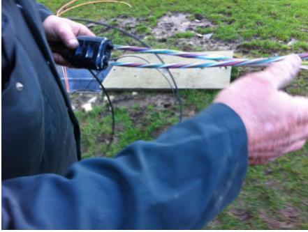
Outer sheath of the fibre removed.
