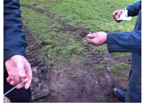
Tube sheath of the fibre removed.
