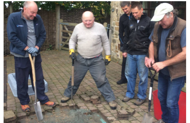
Digging the chamber.
