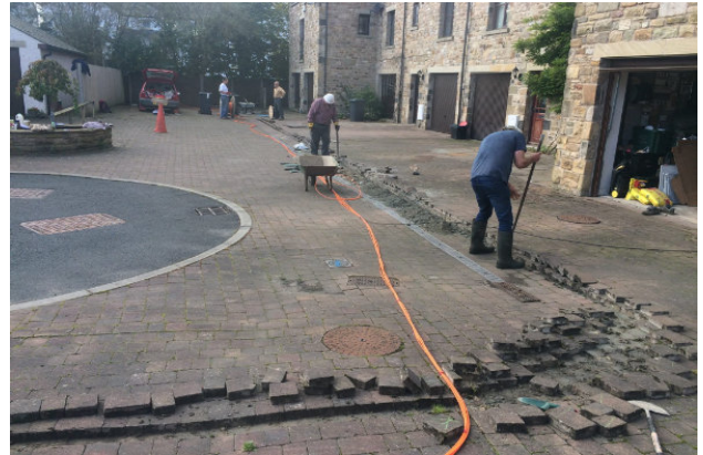
Digging out the trench.
