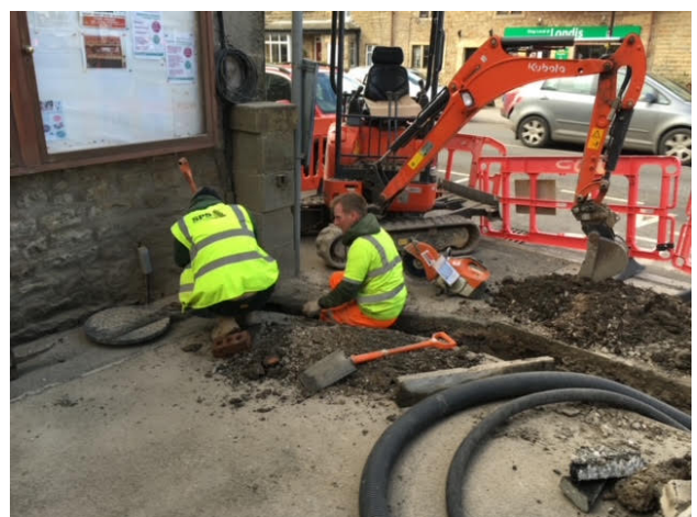
Duct laid under the pavement in sub ducts.
