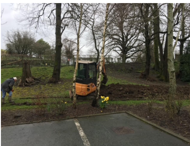
Dave working with the digger man.
