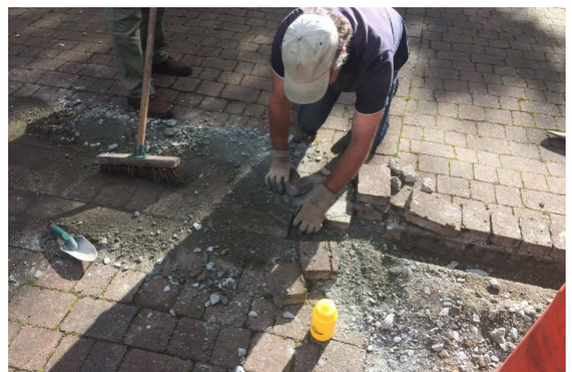
Chris re-instating the cobbles after a dig in Arkholme.
