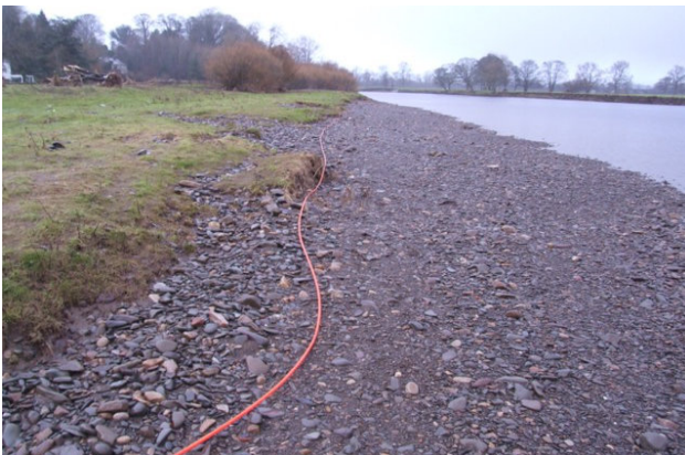
The broken duct beached.
