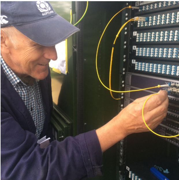
Graham patching customers.
