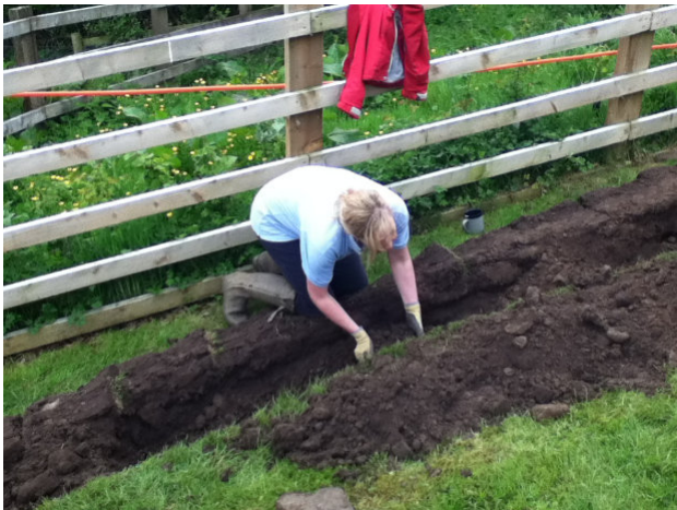
Putting soft fill on the duct.
