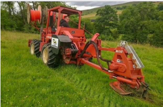
Pneumatic mole plough in action.
