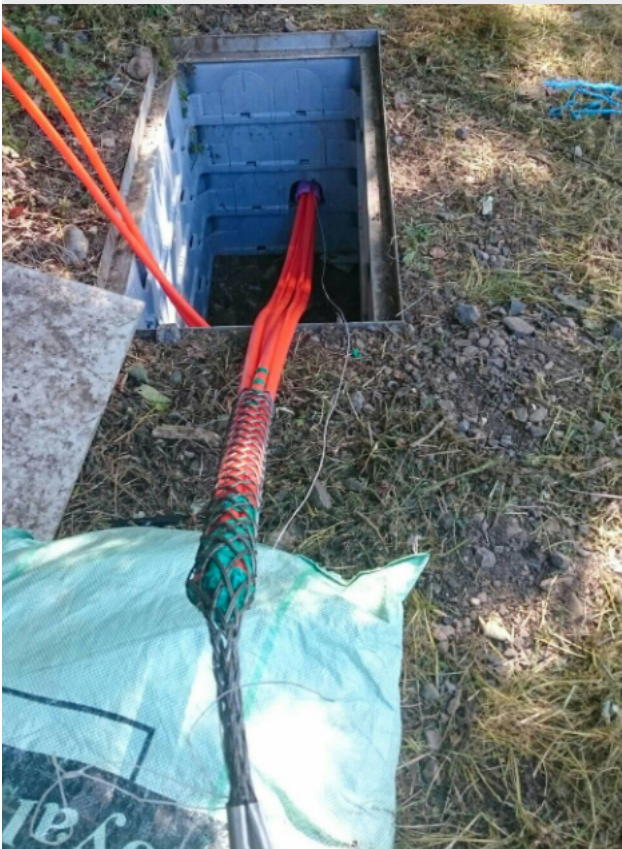
Pulling duct into a chamber, 'One heck of a tight fit'.
