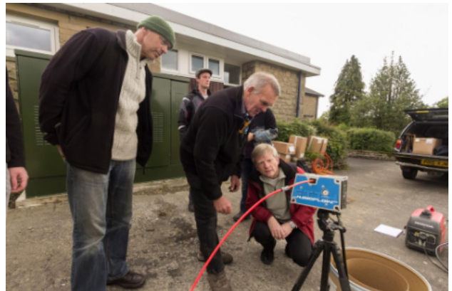
Frank showing the volunteers how the nano flow blower works.
