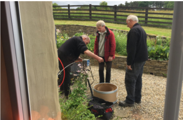
Will Dehany and Frank Brown blowing house fibres.
