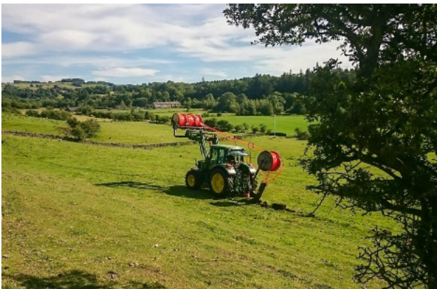
Contractor laying duct with his self-built mole plough.
