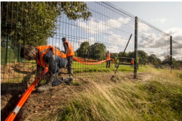
Team at work laying multiple ducts.
