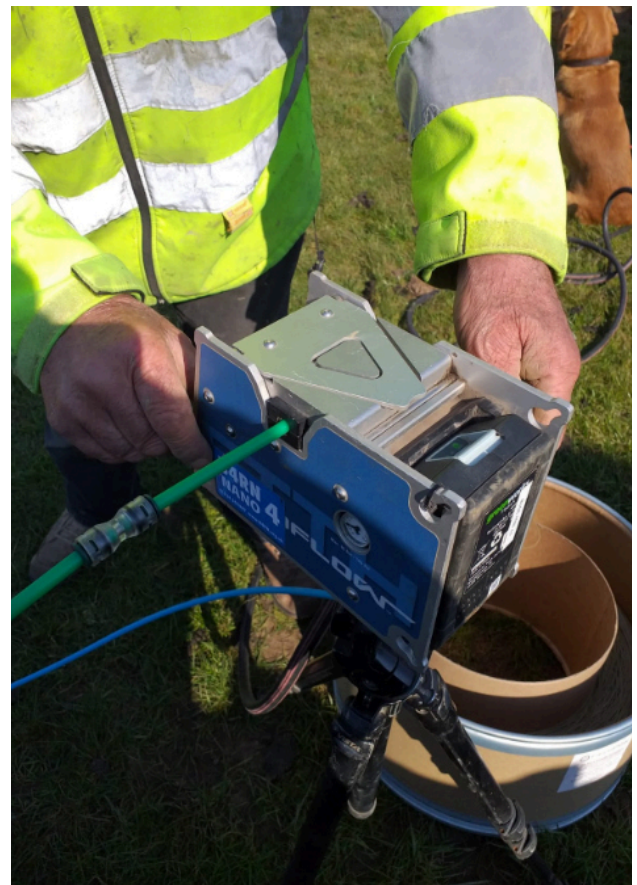
Frank blowing house fibre.
