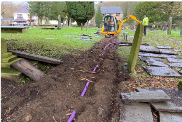
Subduct being used under the flagstones.
