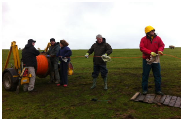
The Wray and Lowgill towel volunteers blowing the fibre over Littledale.
