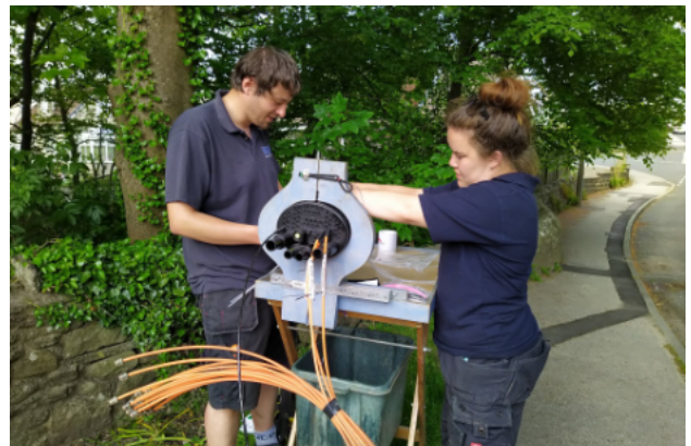
Rob Staveley and Lucy Hawkins working on a large bullet on Caton Road.
