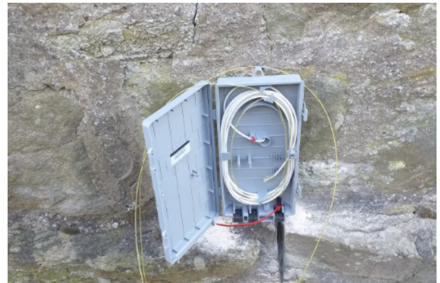
House fibre blown into the outside box ready to fuse.
