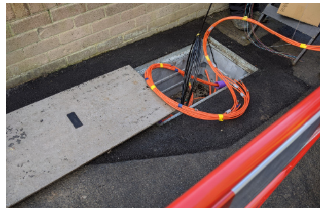
A chamber with ducts and fibre.
