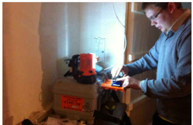
Alistair fusing the house connection.
