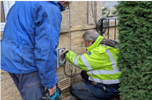
Fitting an external house kit.
